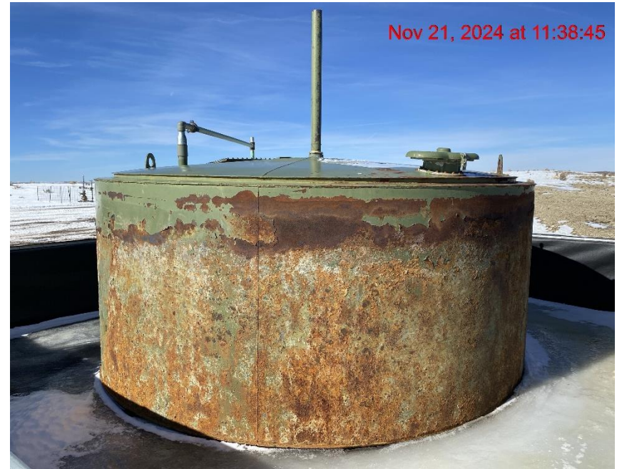
Tank Not Labeled/Corroding Paint – Photo #05048
