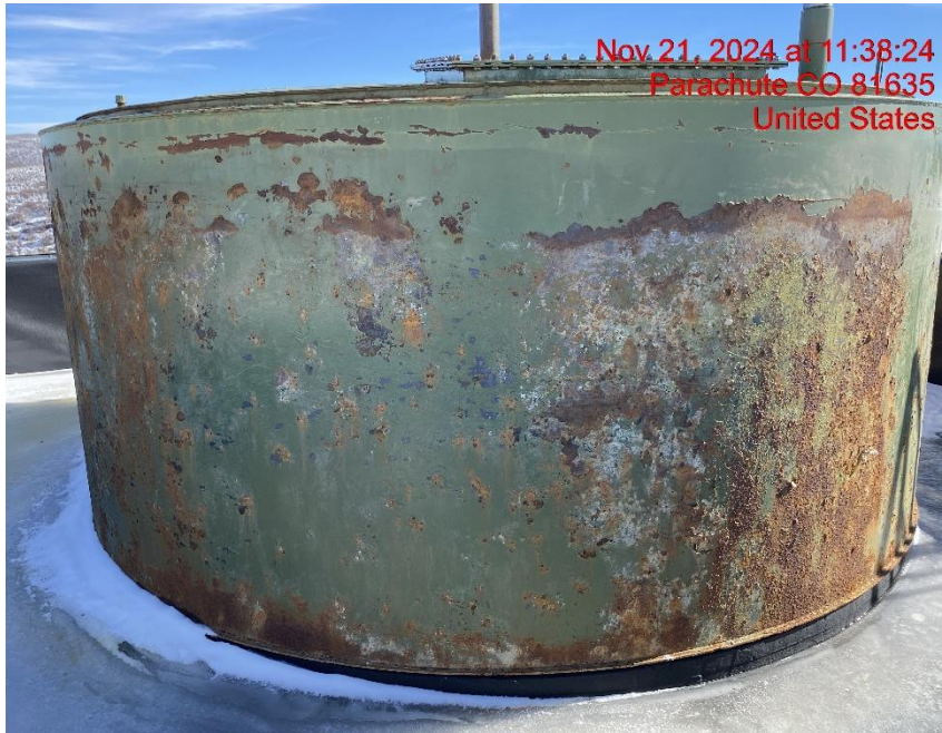
Tank Not Labeled/Corroding Paint – Photo #05047
