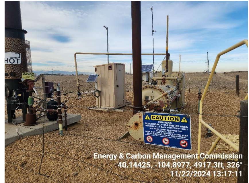
Photo 6 ECD, Gas Meter Run & Horizontal Heated Separator.
