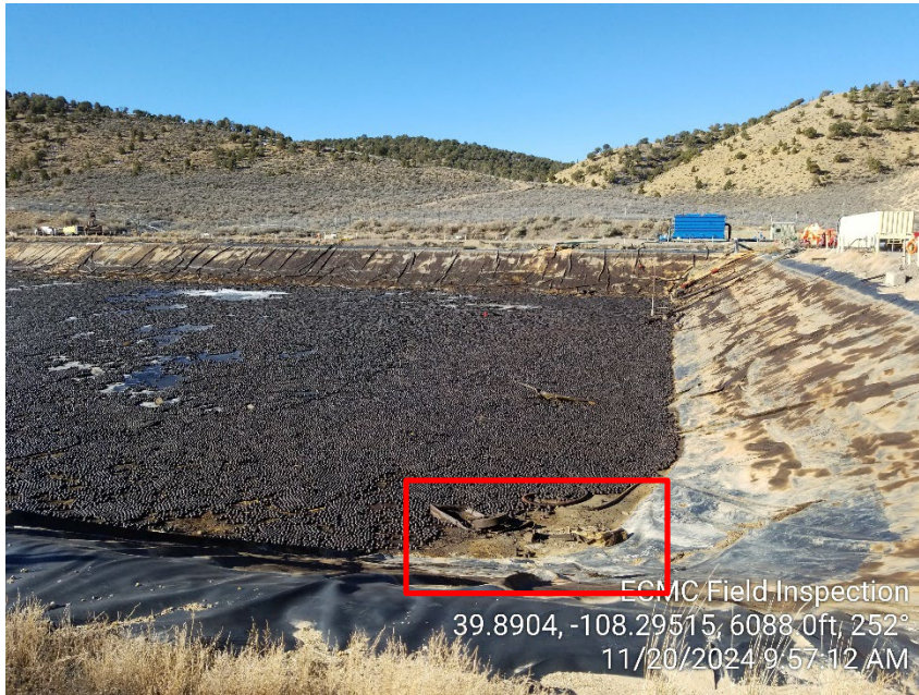
Photo #3 – Overview of pit from east, note debris and equipment (hoses) present on liner in northeast corner.
