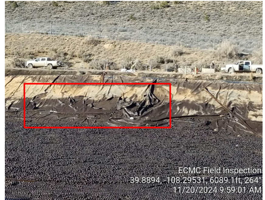
Photo #4 – Damaged section of liner in SW corner of pit.
