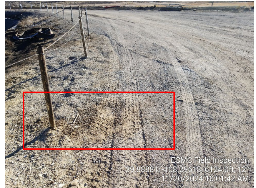
Photo #8 - Stained soil (E&P Waste) located on pit berm (4).
