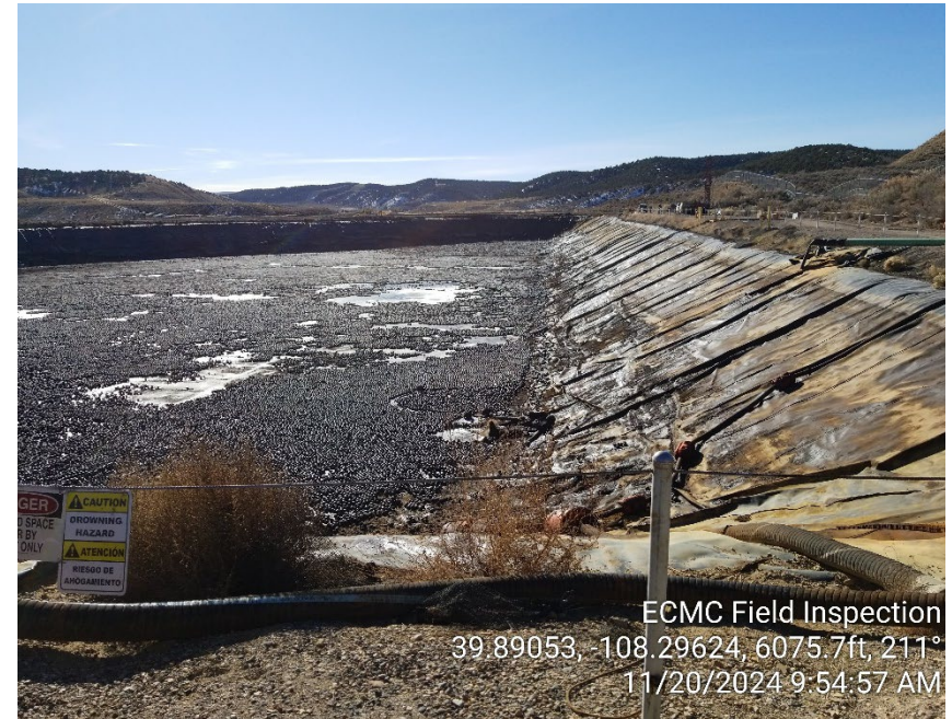
Photo #2 – Overview of pit from the north. Note: hydrocarbons observed on pit liner.
