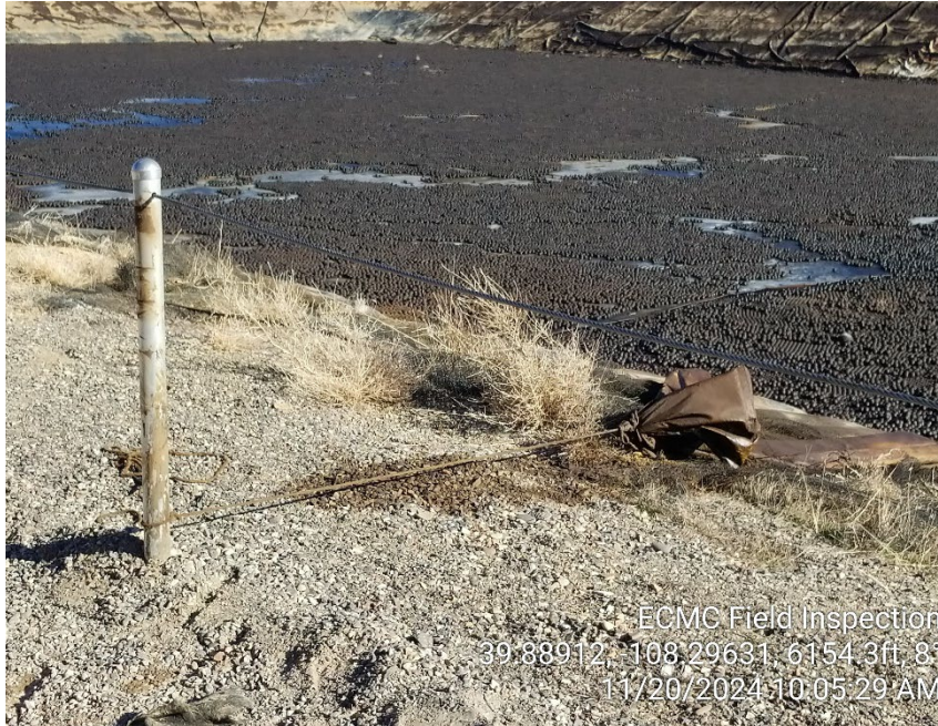
Photo #7 - Stained soil (E&P Waste) located on pit berm (3).
