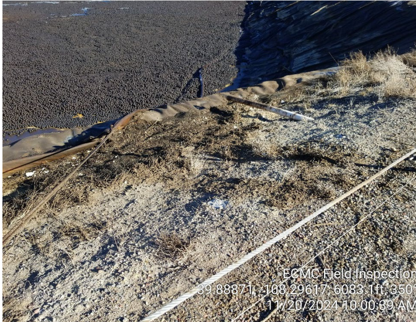
Photo #5 – Stained soil (E&P Waste) located on pit berm (1).
