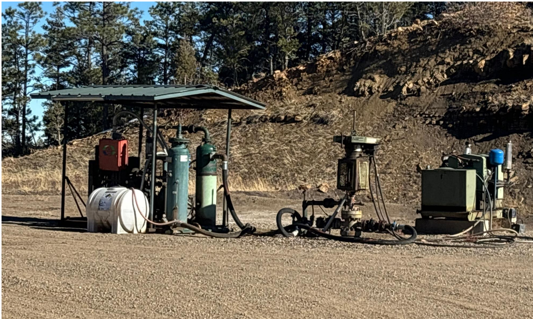
PHOTO 3: WELLHEAD AND EQUIPMENT.
