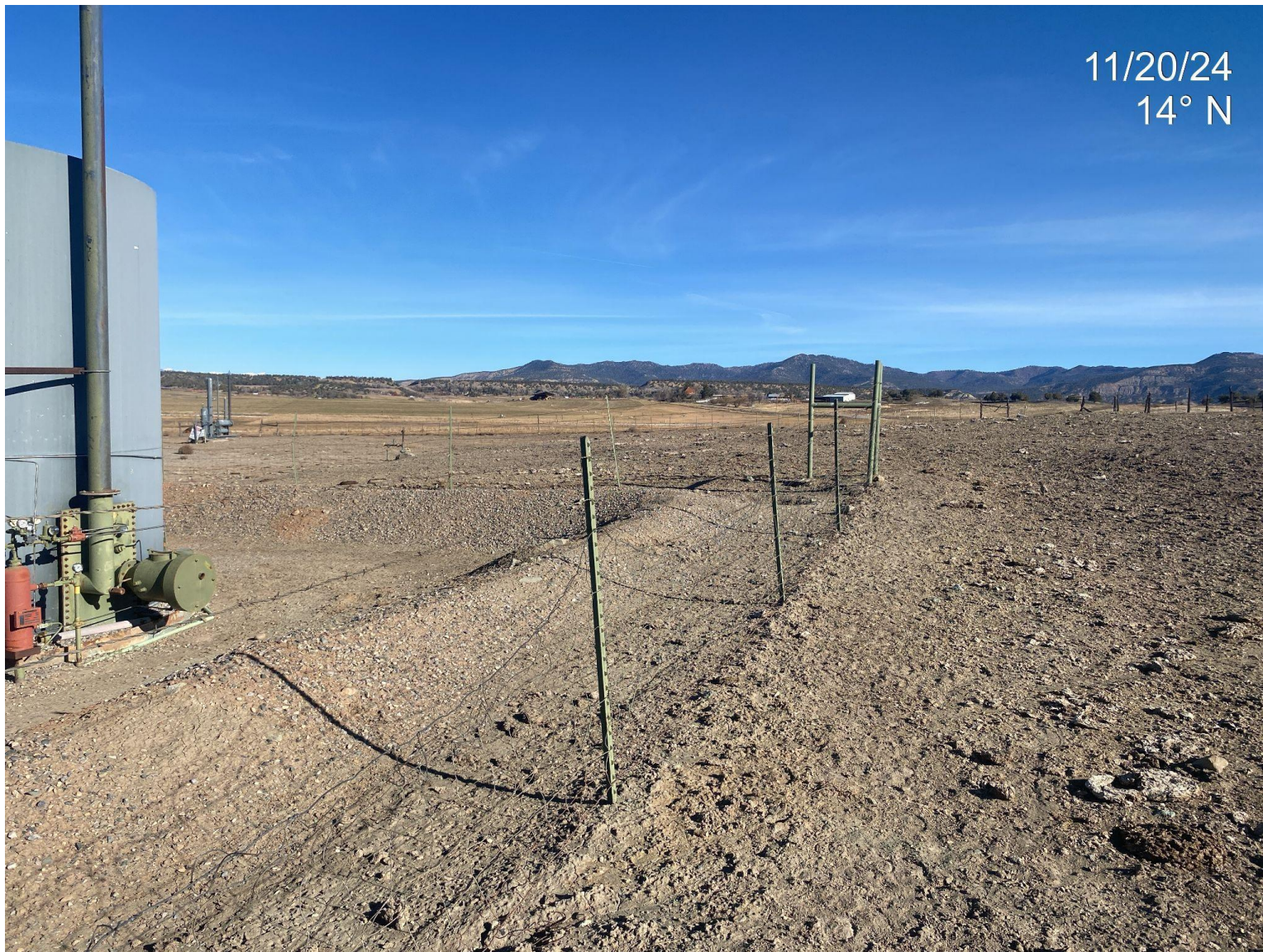
Photo 2. Fence around produced water tank is in working order.
