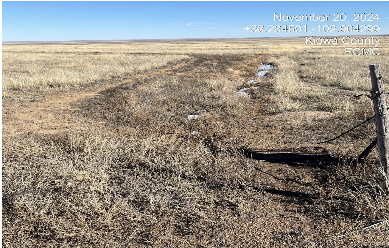
Photo 1. Facing east at the access road. The cattleguard has not been removed and has filled in with sediment. The access road has not been recontoured or reclaimed in this area.
