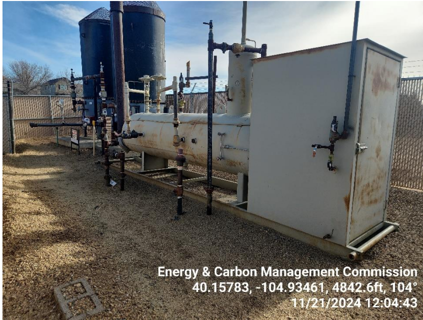
Photo 7 Horizontal Heated Separator.
