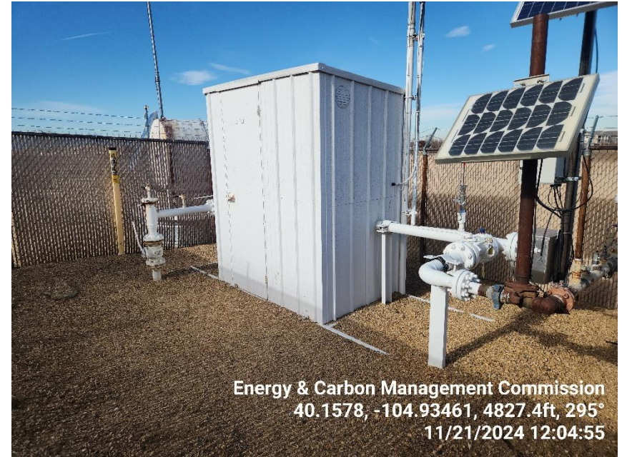
Photo 8 Gas Meter Run.
