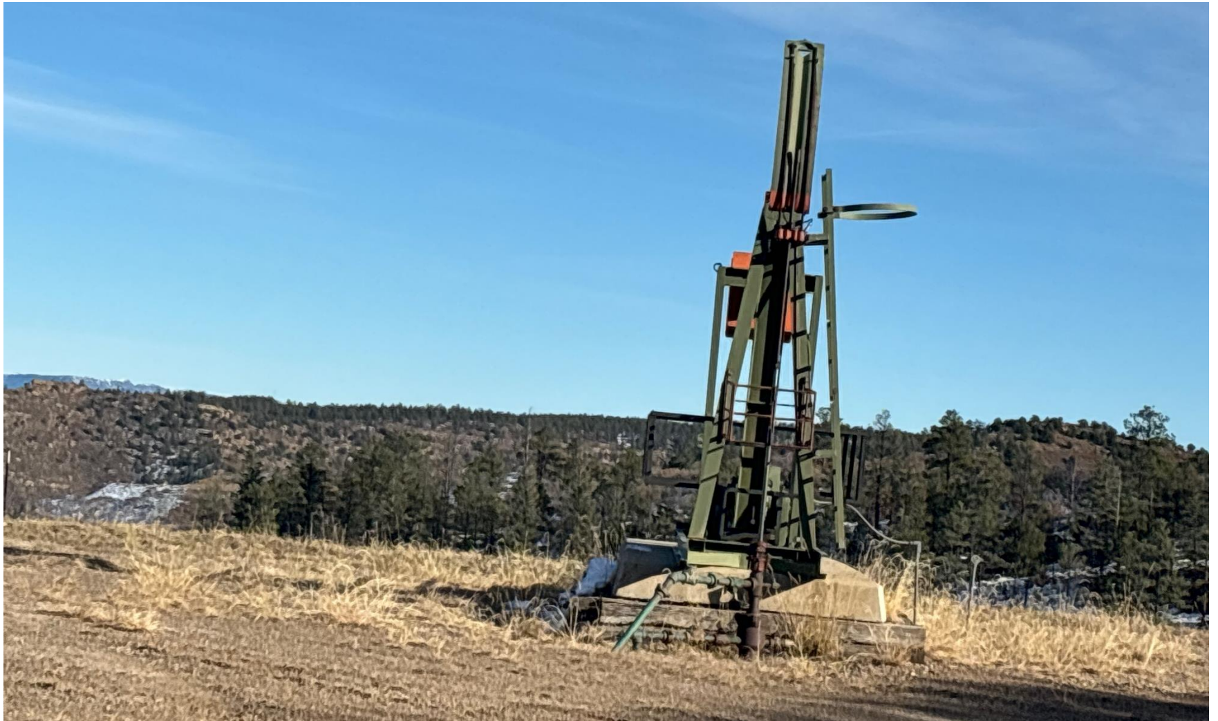
PHOTO 3: WELLHEAD AND EQUIPMENT.
