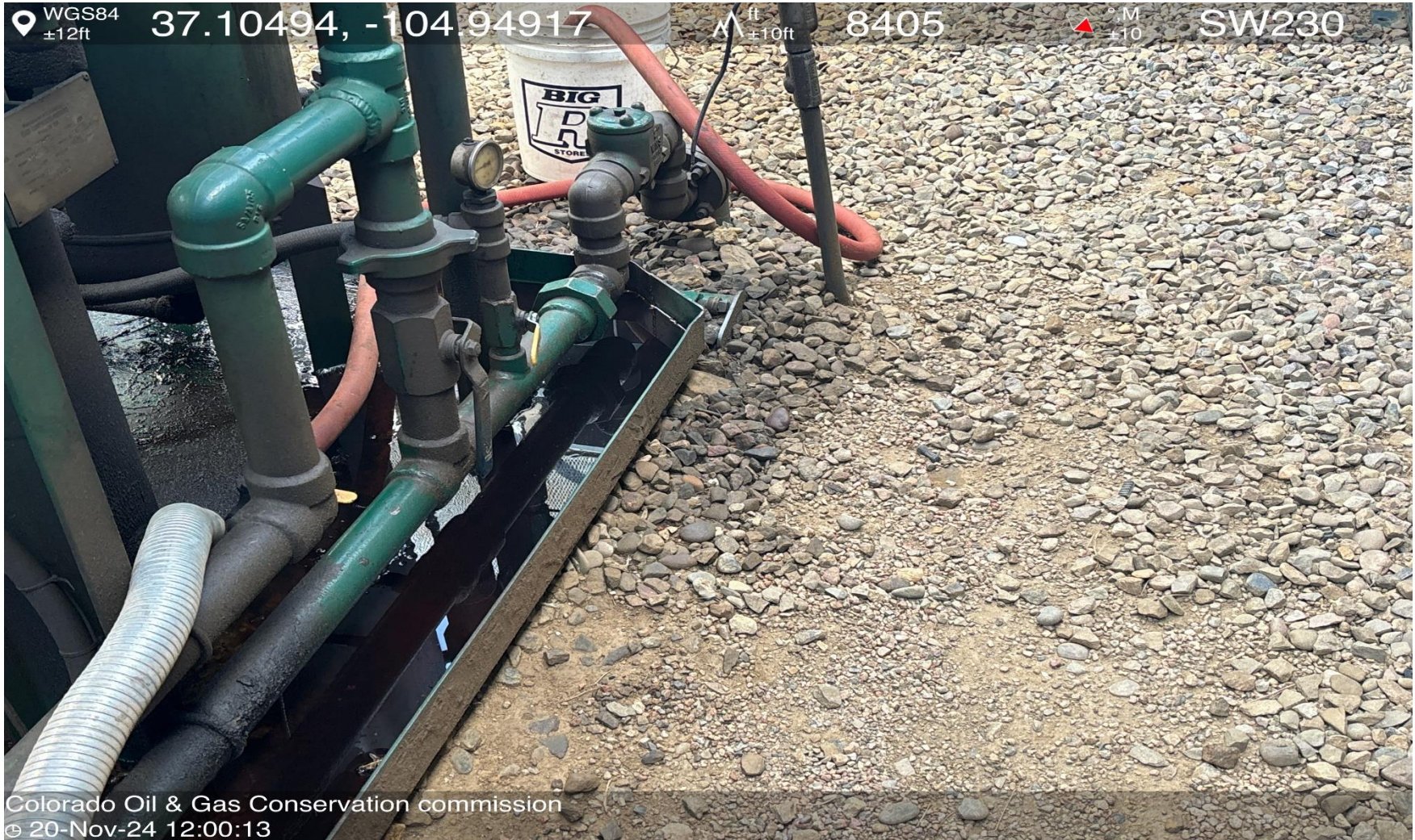
PHOTO 6: AREA OF IMPACTED SOIL NEAR COMPRESSOR. Conduct maintenance on equipment, cleanup stained material and review self inspection processes. COMPLY WITH RULE 1002,(2).D. CA DATE 11/30/2024.
