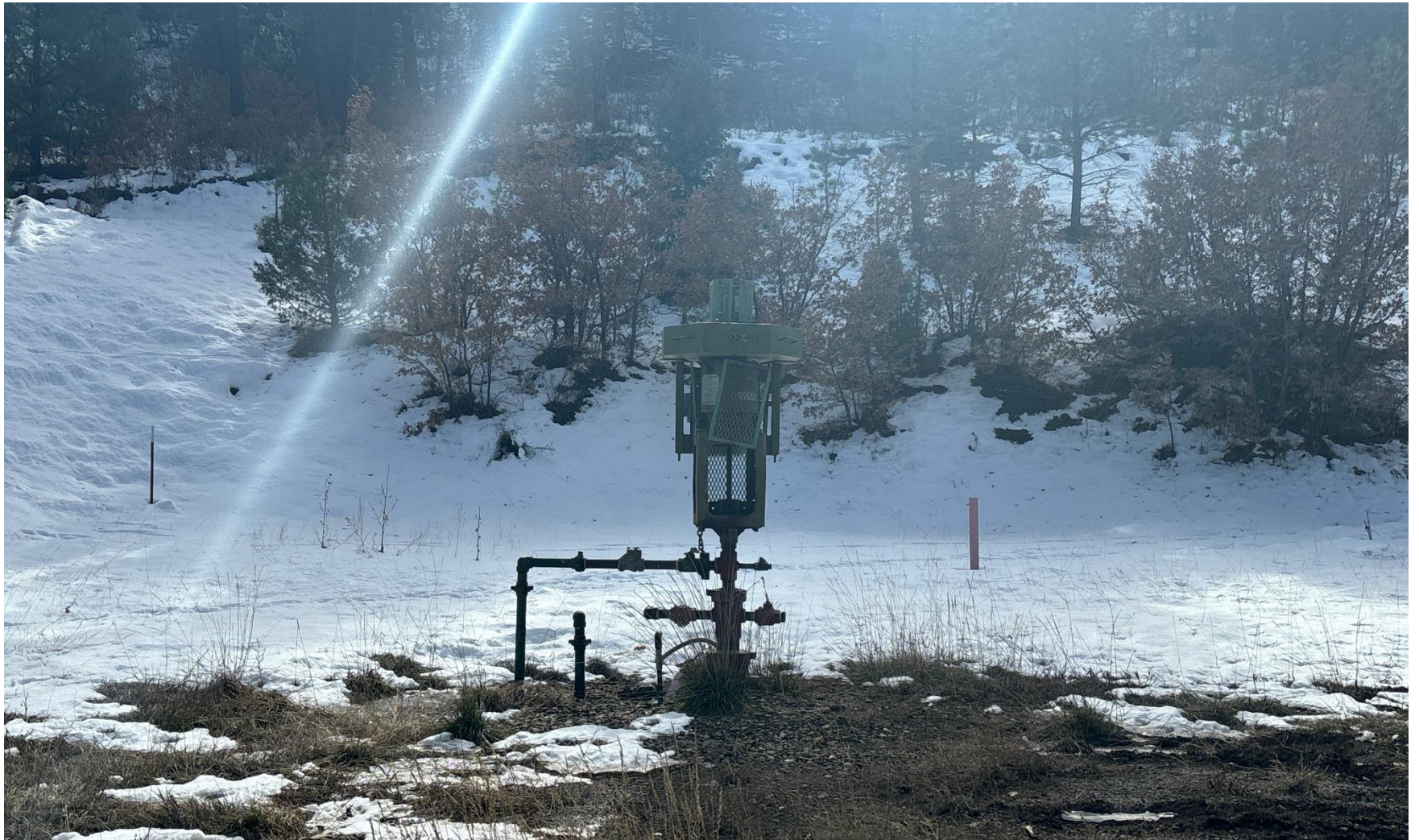
PHOTO 3: WELLHEAD AND EQUIPMENT.
