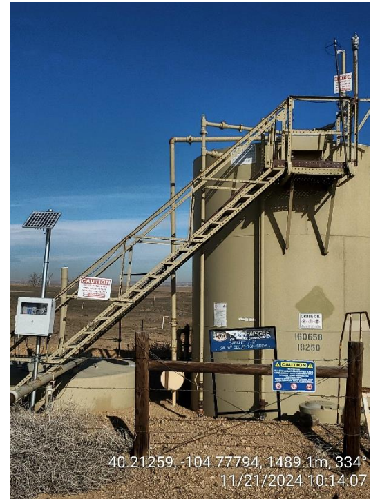
Battery on East Side
