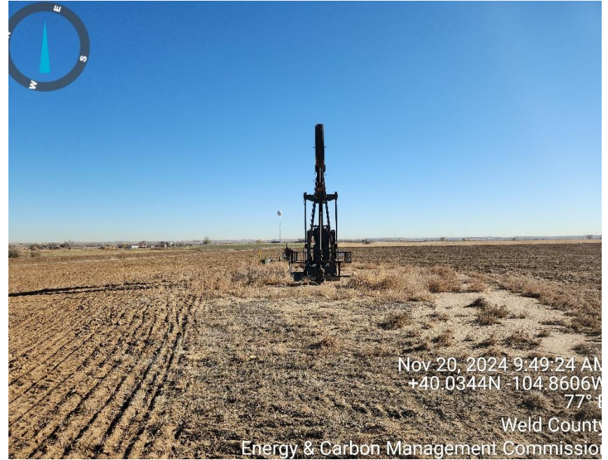
Photo 2 well head and equipment
