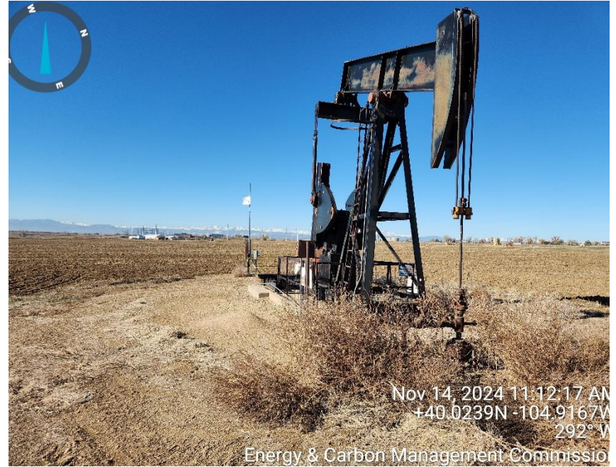
Photo 2 well head and equipment
