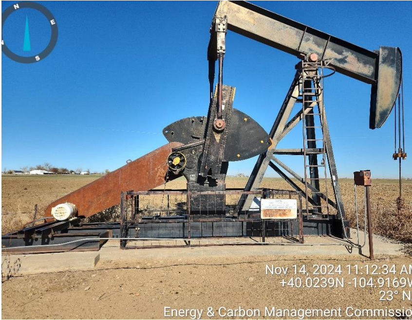
Photo 1 well head and equipment
