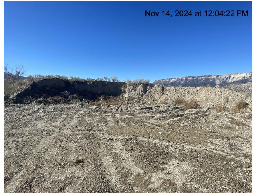
Photo # 9988 Stored stockpile on location (additionally stockpiled materials lack Stormwater BMP's & stockpile is interfering with interim reclamation)
