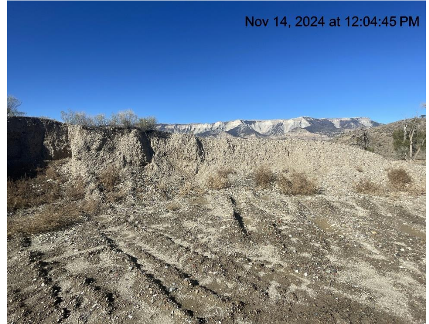
Photo # 9990 Stored stockpile on location (additionally stockpiled materials lack Stormwater BMP's & stockpile is interfering with interim reclamation)
