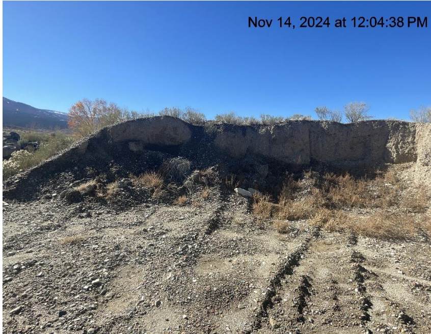
Photo # 9989 Stored stockpile on location (additionally stockpiled materials lack Stormwater BMP's & stockpile is interfering with interim reclamation)
