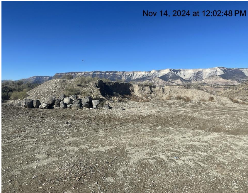
Photo # 9987 Stored stockpile on location (additionally stockpiled materials lack Stormwater BMP's & stockpile is interfering with interim reclamation)
