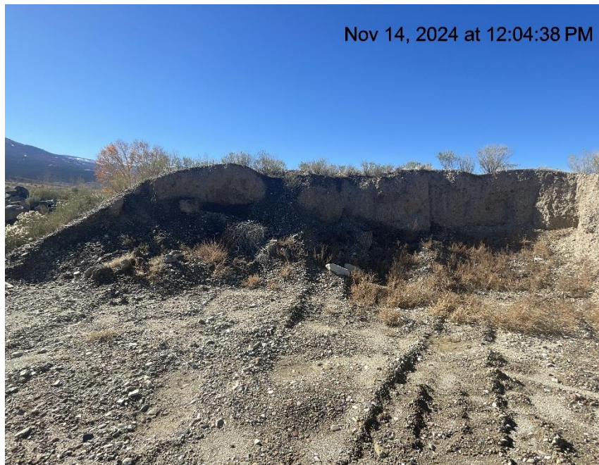
Photo # 9993 Stockpile lacks BMP's
