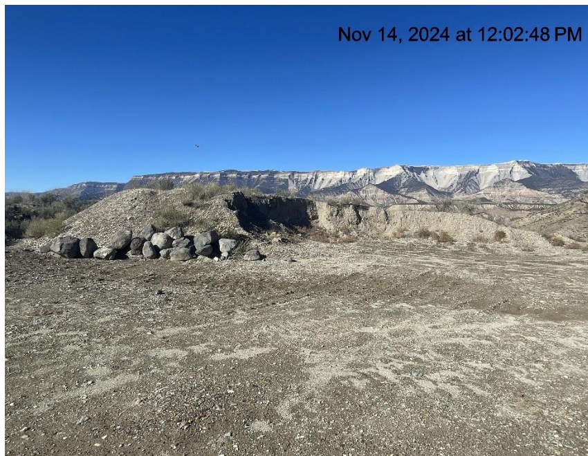
Photo # 9991 Stockpile lacks BMP's
