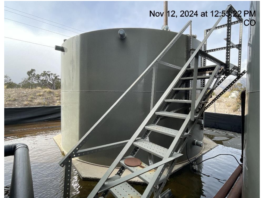
Photo # 9900 Tank lacks required labeling
