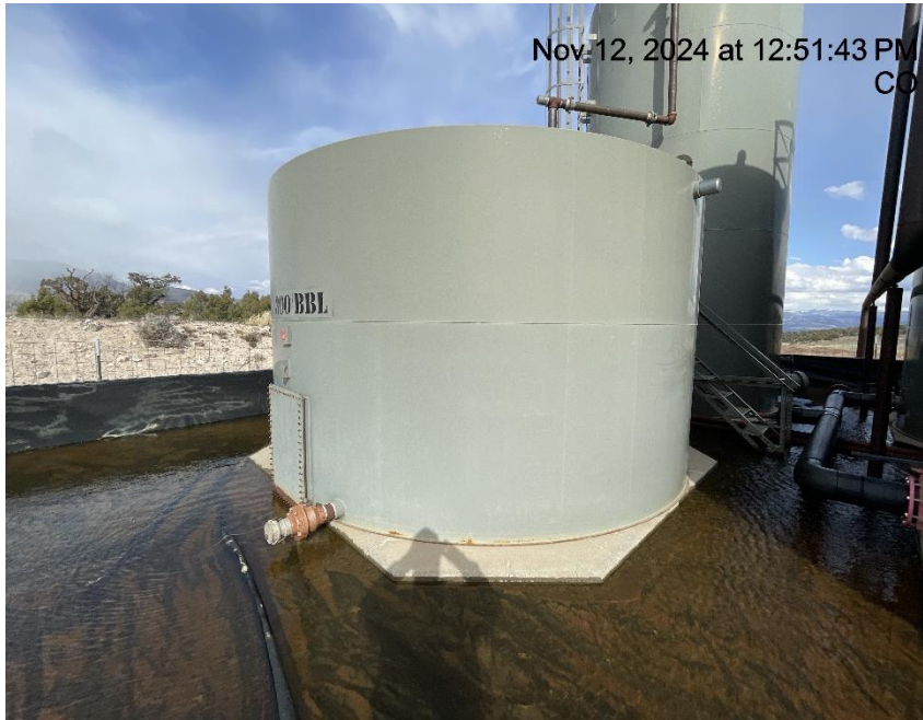
Photo # 9897 Tank lacks required labeling
