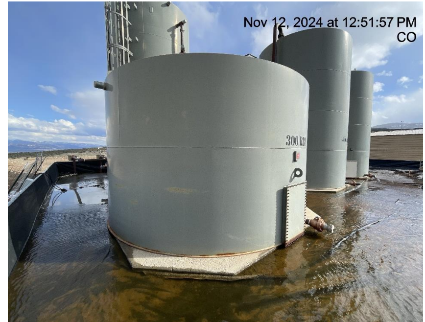
Photo # 9898 Tank lacks required labeling
