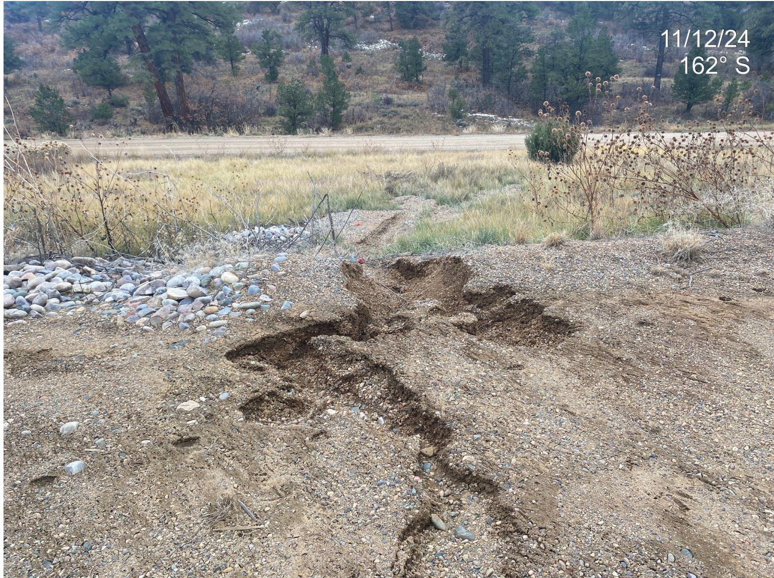
Photo 3. Gully erosion on the southern edge of the pad.
