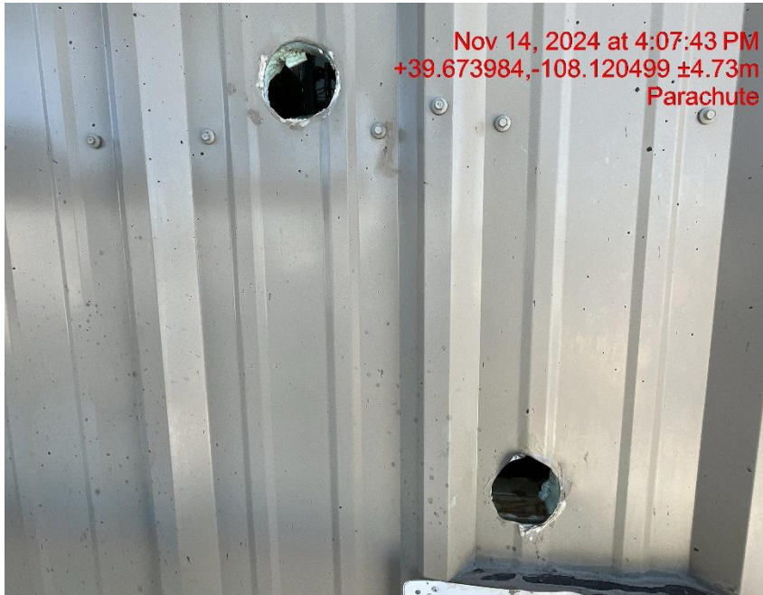
Photo # 9236 Open holes on gas meter building/wildlife hazard available for entry by wildlife
