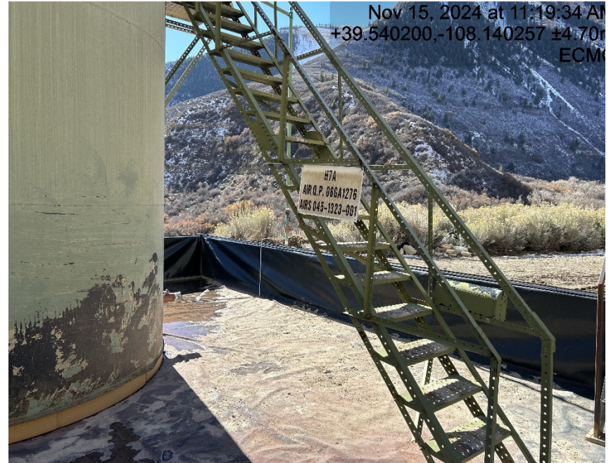
Lack of proper battery signage
