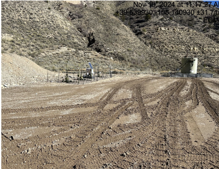
Location and lack of stabilization/compaction
