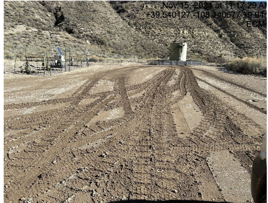
Location and lack of stabilization/compaction
