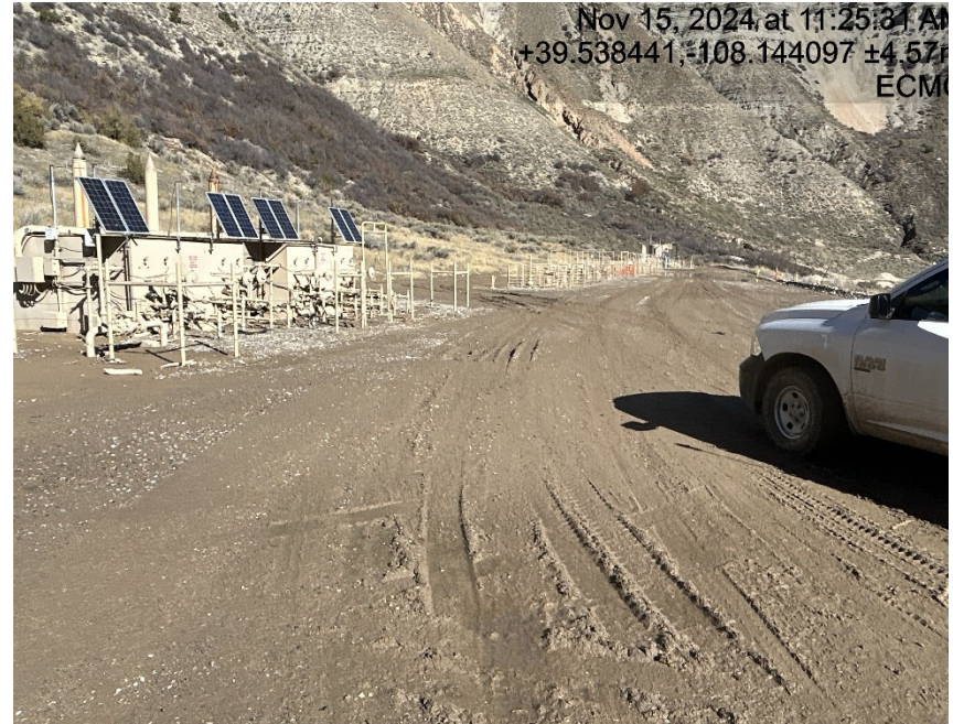
Location and Lack of stabilization/ compaction
