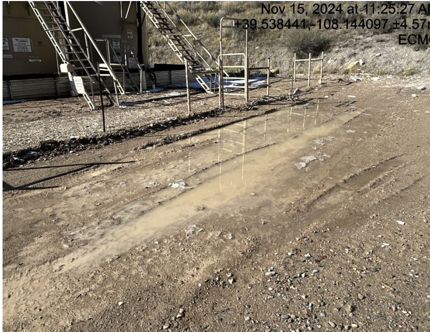
Lack of stabilization/ compaction
