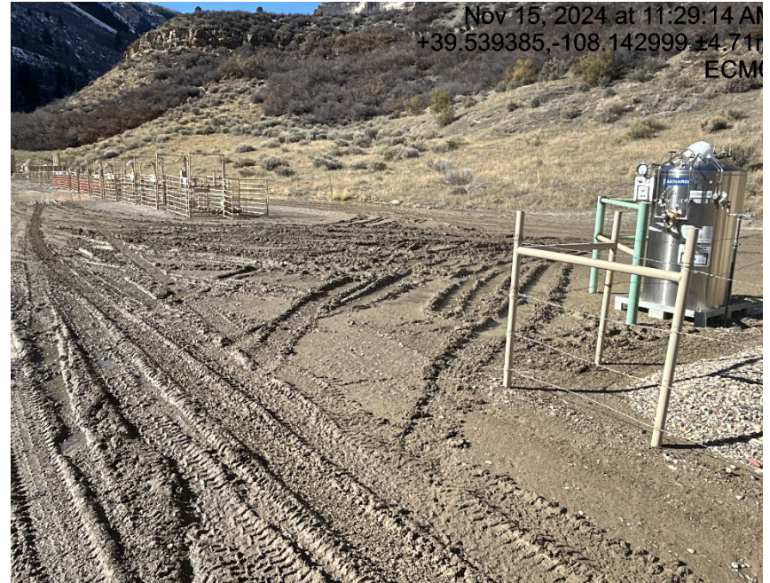
Lack of stabilization/ compaction
