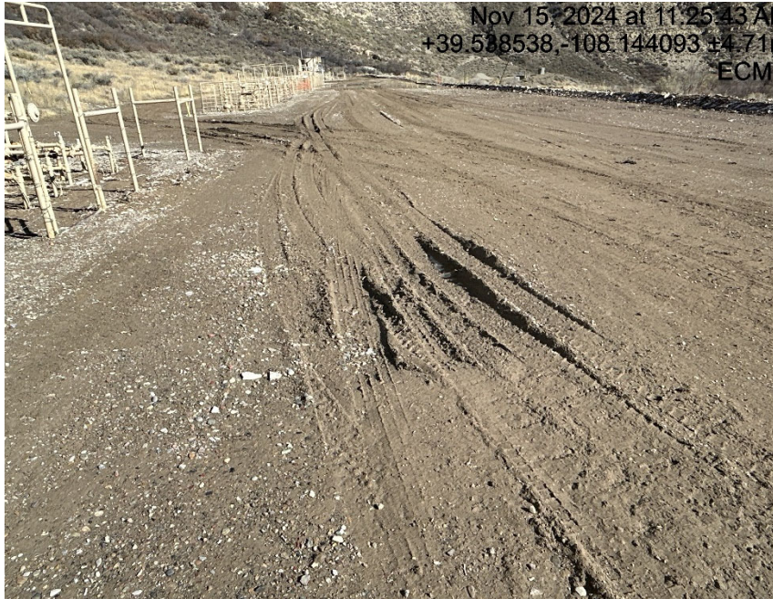
Lack of stabilization/ compaction
