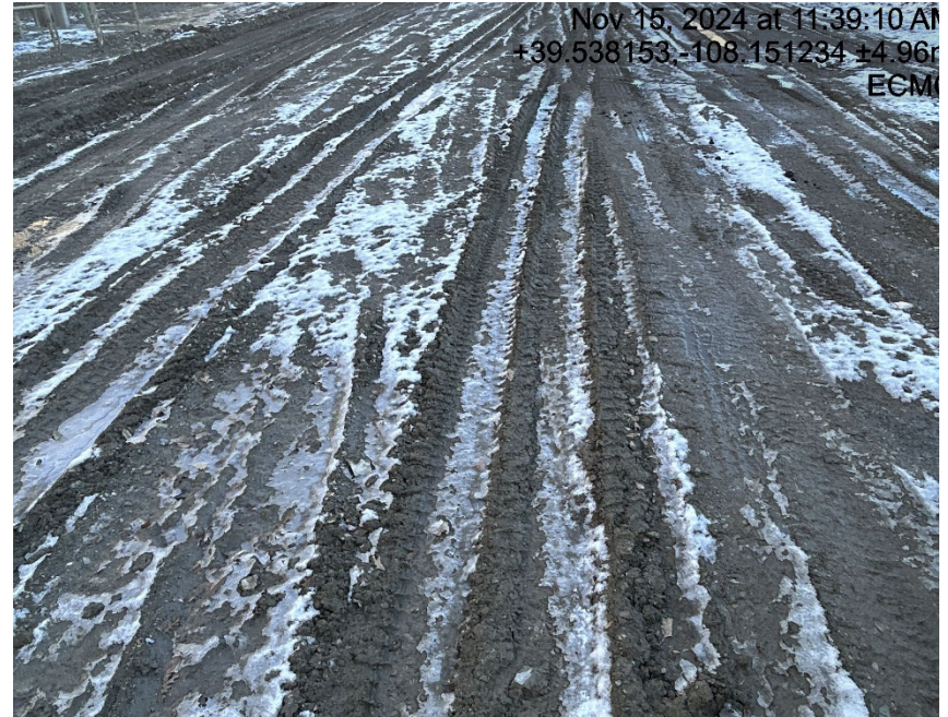
Lack of stabilization/compaction
