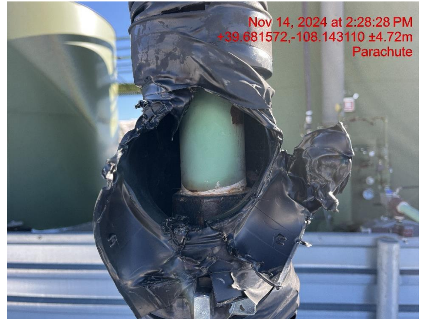
Photo # 9182 Flow line heating insulation open ended/wildlife hazard available for entry by wildlife
