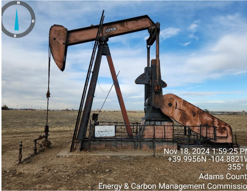
Photo 1 well head and equipment
