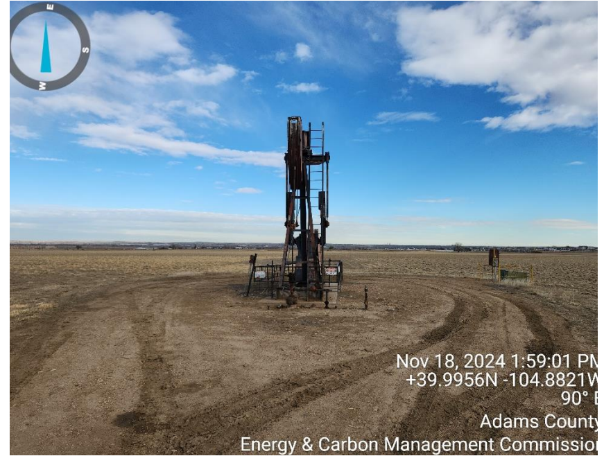
Photo 2 well head and equipment
