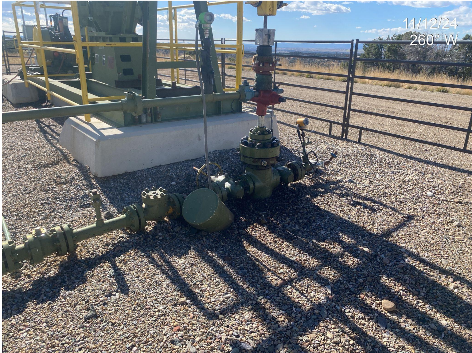
Photo 3. Impacted surface material has been removed from around well head.
