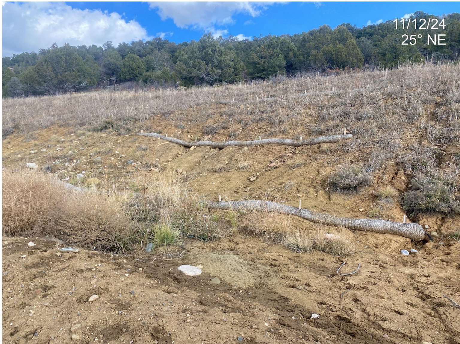
Photo 3. Stormwater BMPs have been installed in the northern portion of the location.
