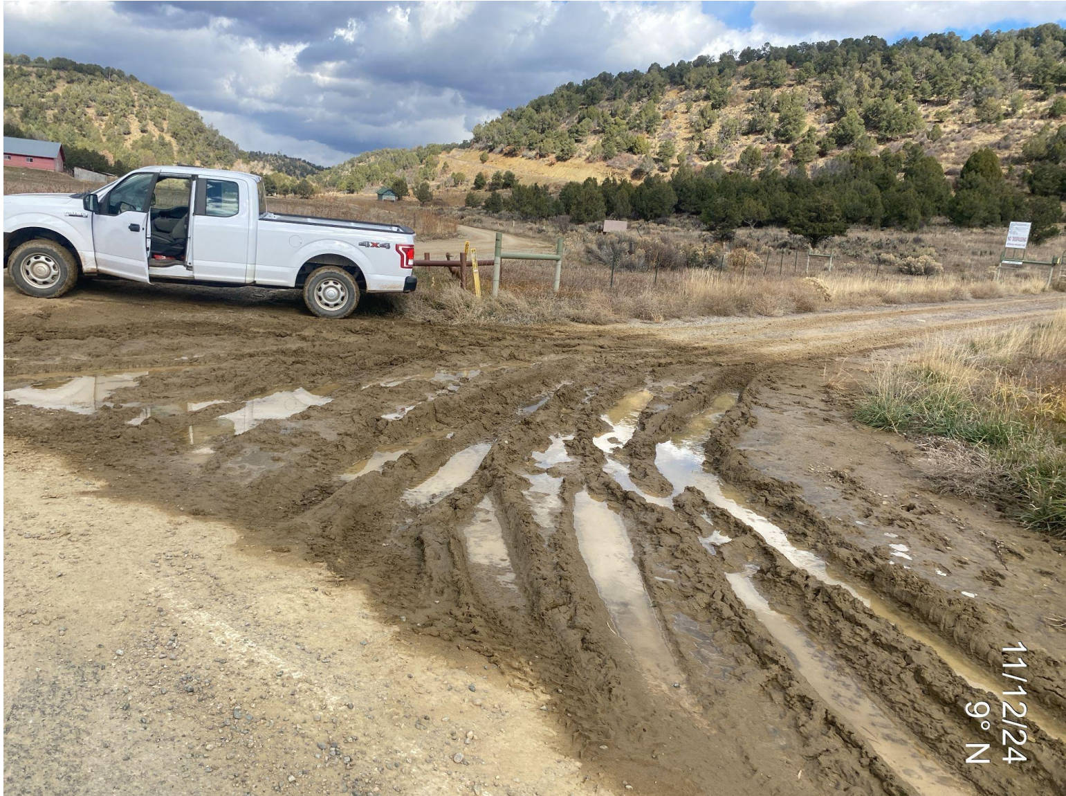
Photo 5. Severe rutting observed at access point. Additional stabilization/grading needed to minimize degradation to access point.
