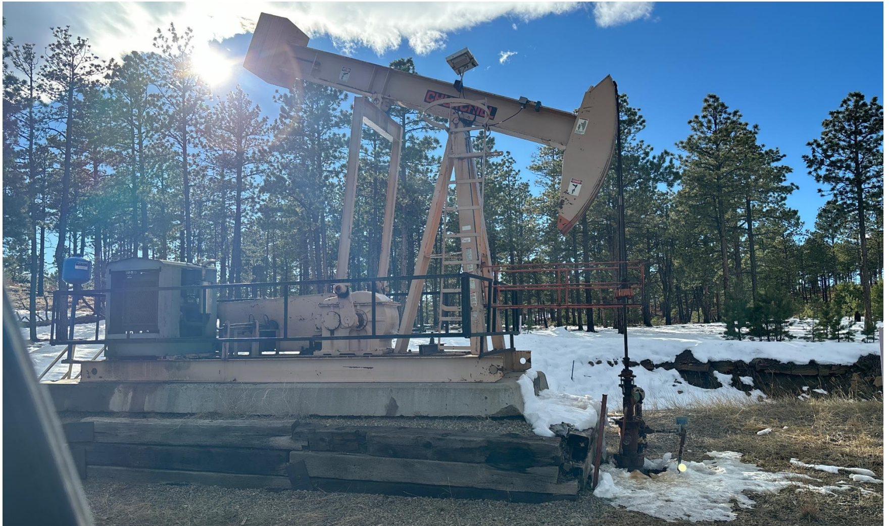
PHOTO 3: V WELLHEAD AND EQUIPMENT.
