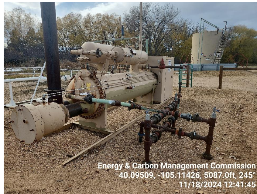
Photo 4 Horizontal Heated Separator.
