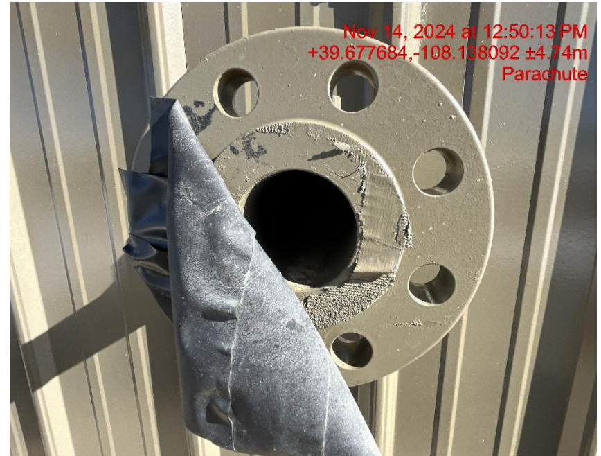
Photo # 9073 Open ended piping/wildlife hazard/ available for entry by wildlife
