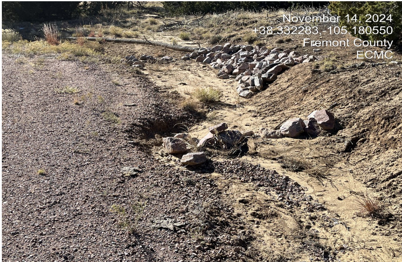
Photo 2. There are check dams where stormwater has eroded around the check dam. BMP maintenance is required.
