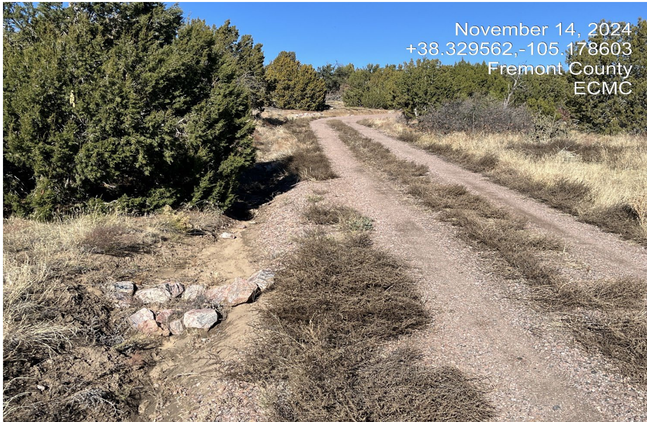
Photo 1. Facing northwest along the access road. There are check dams that are filled in and not maintained and erosion along the roadside.
