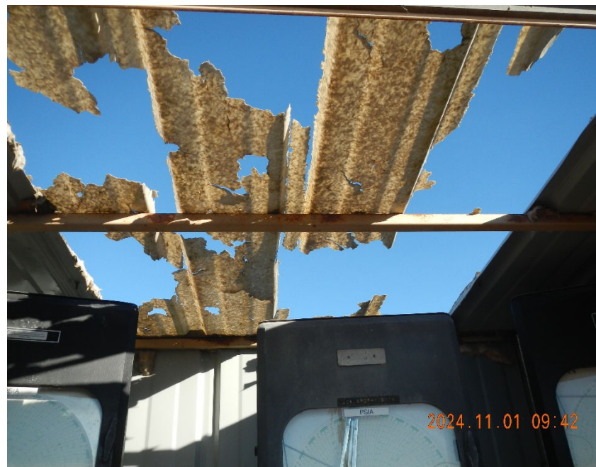
8. View of meter shed roof damage.
