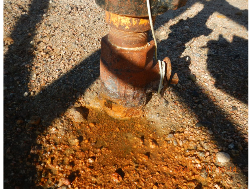
4. Valve on water leg that is leaking produced water.
