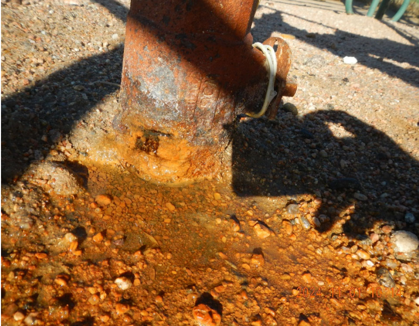
5. View of base of valve where leak is originating.
