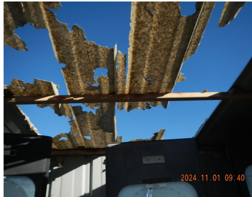
10. Damaged roof on meter shed.
