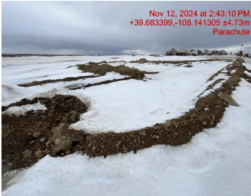
Photo # 9020 Unused berm not compacted and damaged
