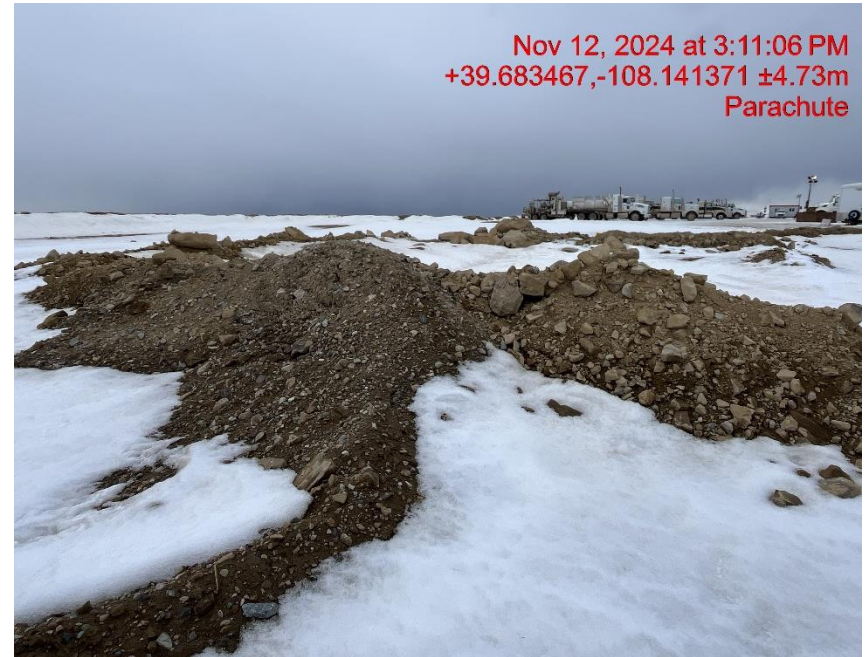
Photo # 9041 Unused berm not compacted and damaged
