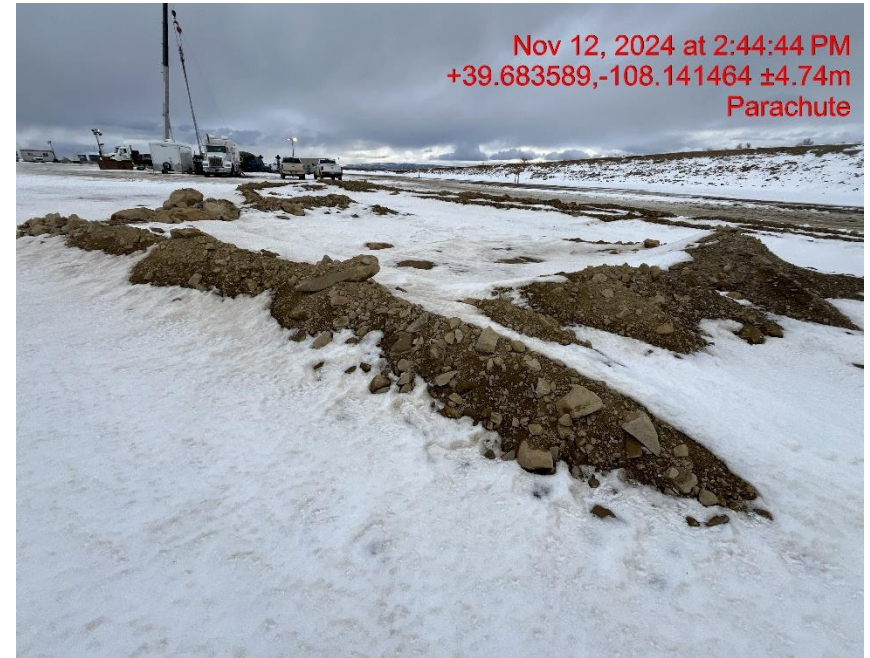
Photo # 9022 Unused berm not compacted and damaged
