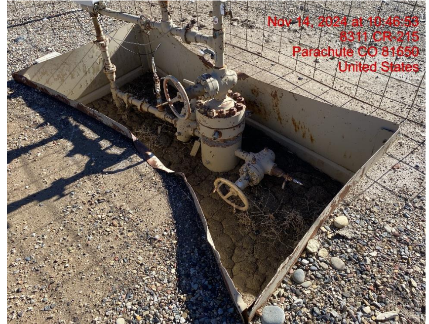
Open Wellhead Cellar/No Wildlife Egress – Photo #04895
