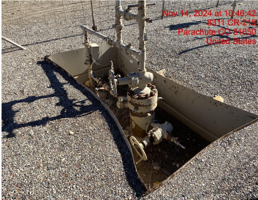
Open Wellhead Cellar/No Wildlife Egress – Photo #04894
