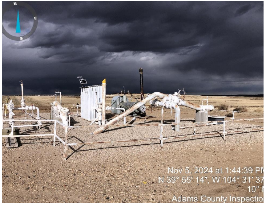
Photo #2 Meter & Separator.
