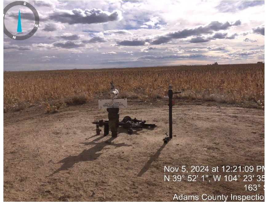
Photo #4 Well head.
