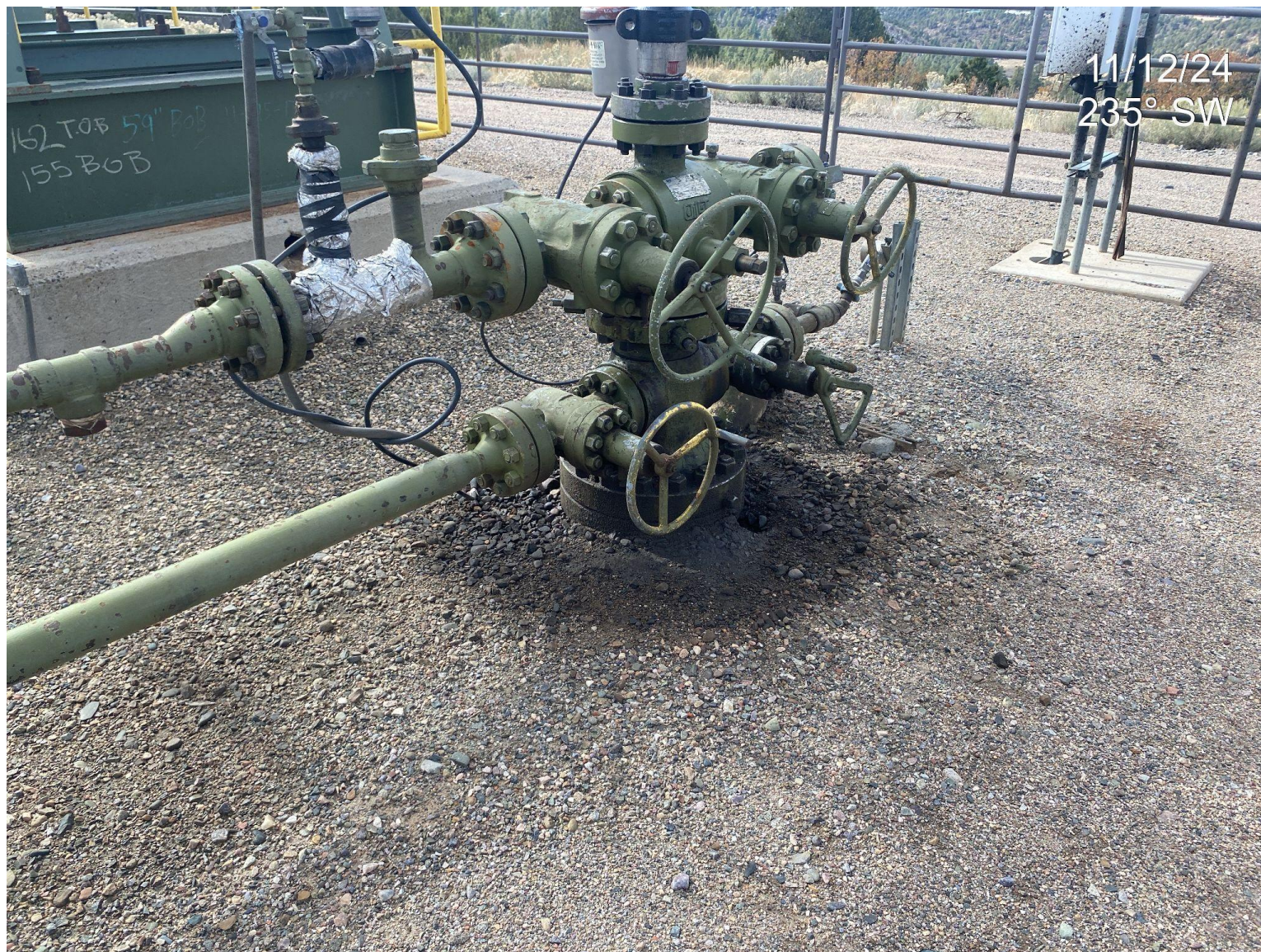
Photo 3. Impacted surface material observed at well head.
