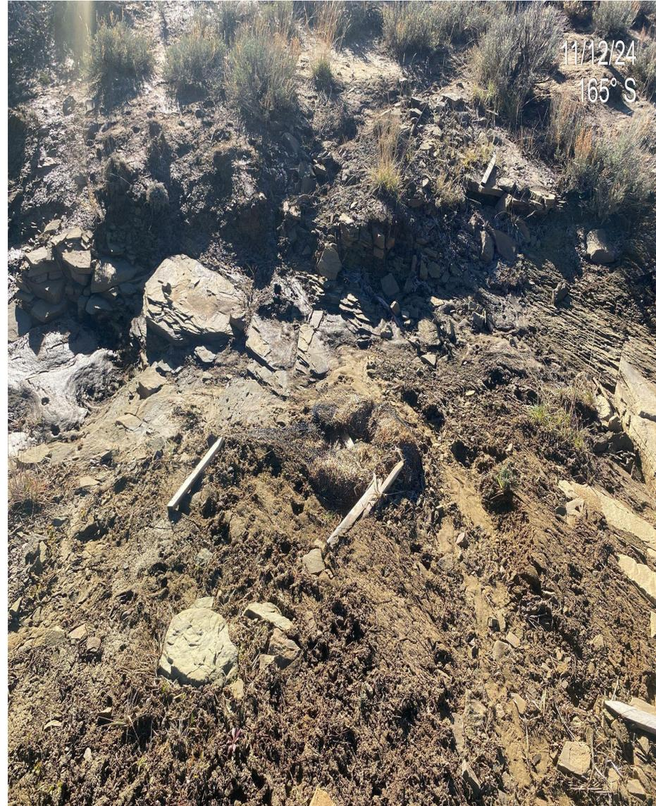
**Photo 2.** Wattles installed in the southeast corner to address erosion issues have not been installed per good engineering practice. Stormwater persists and water is running under the wattles.
