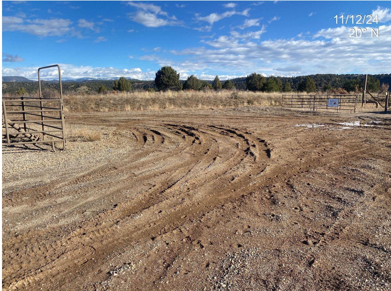
Photo 4. Rutting starting to form on the active pad. Future maintenance/additional stabilization of the active pad is advised.
