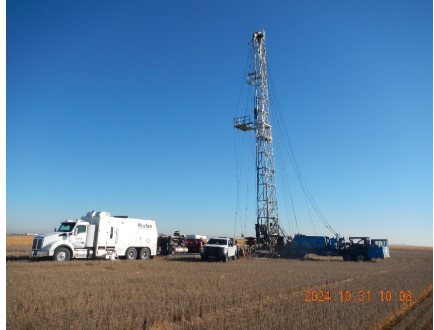
2. View of equipment at well as well plugging and abandonment work is underway.
