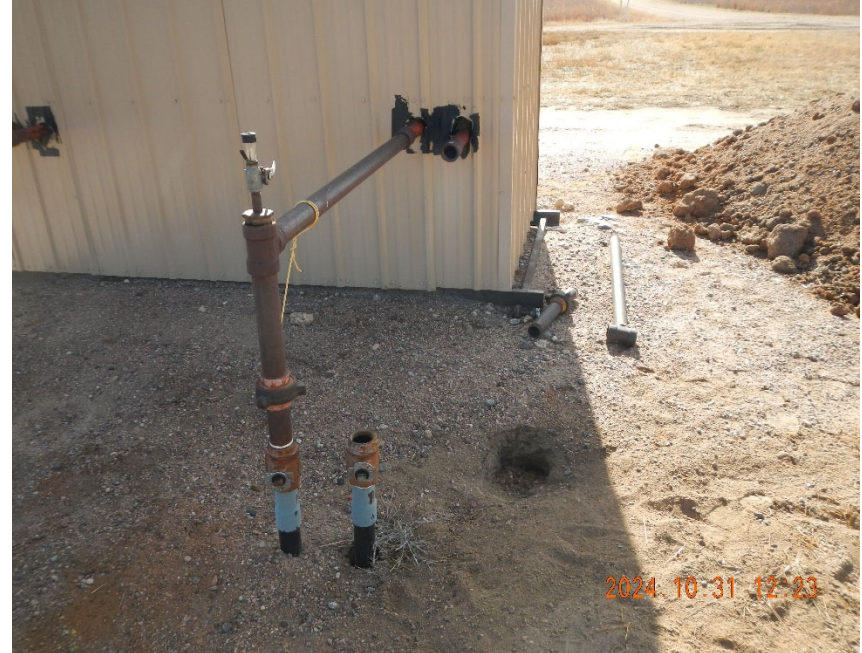
4. View if disconnected and air gapped flowline at remote gather location.
