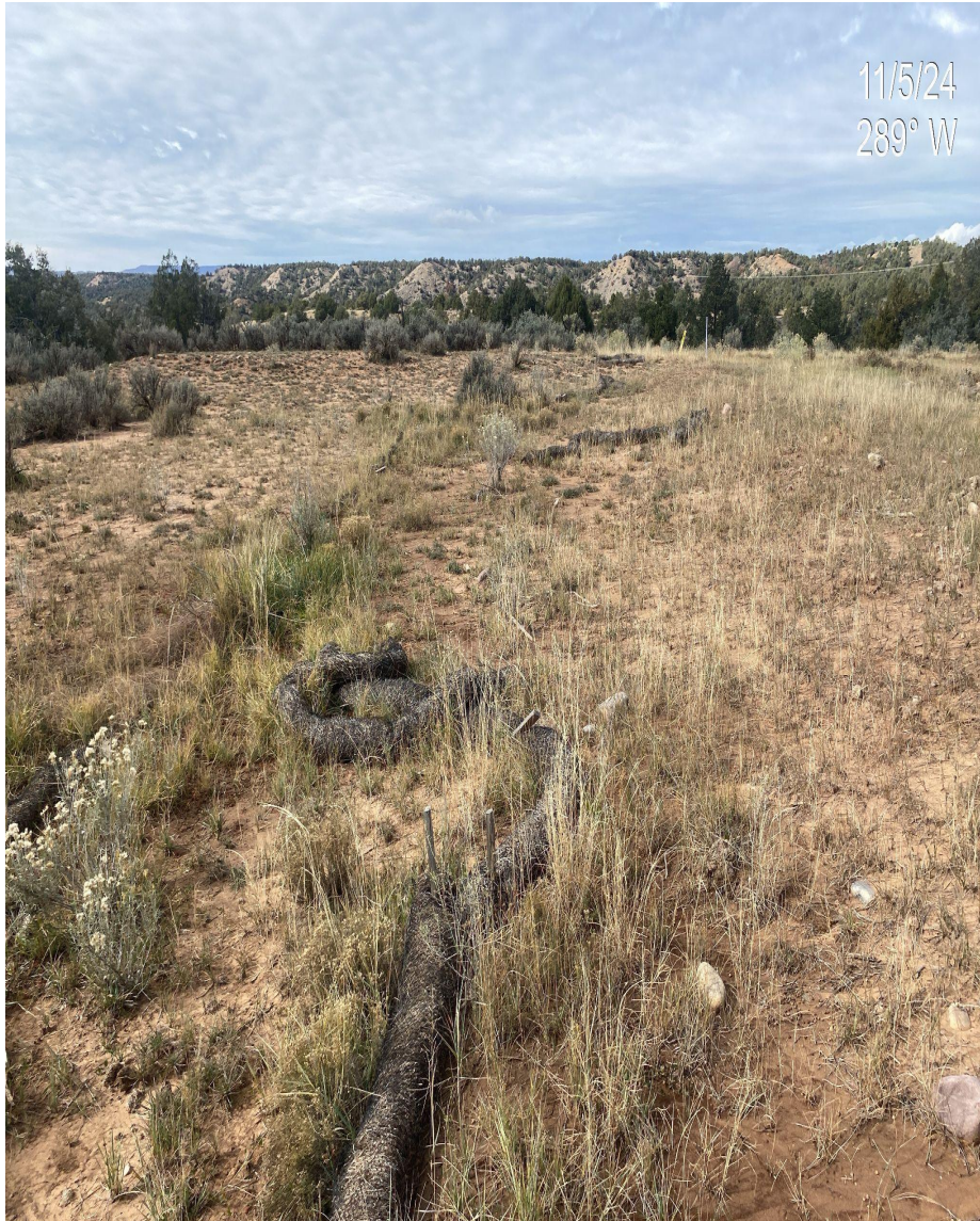
Photo 3. View of stormwater BMP wattles in the southern portion of the disturbance that are not installed correctly and no longer functioning.
