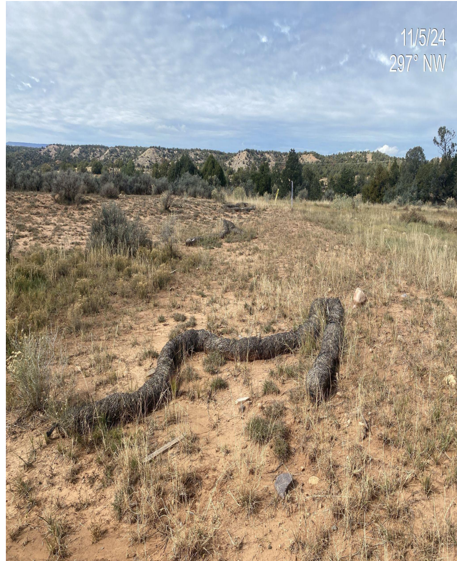
Photo 3. View of stormwater BMP wattles in the southern portion of the disturbance that are not installed correctly and no longer functioning.
