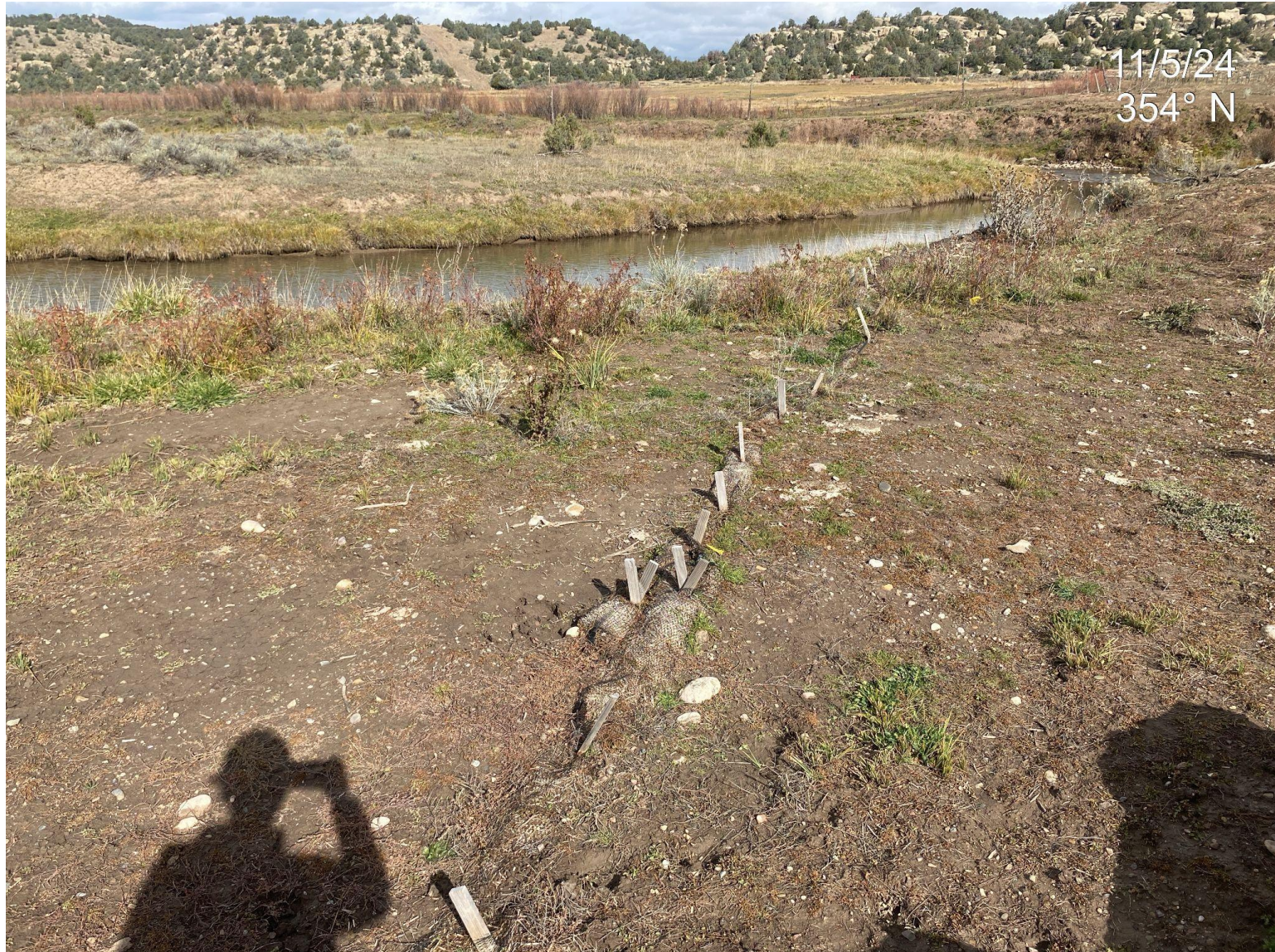
Photo 4. View of stormwater BMP wattles that are filled in with sediment and no longer functioning.
