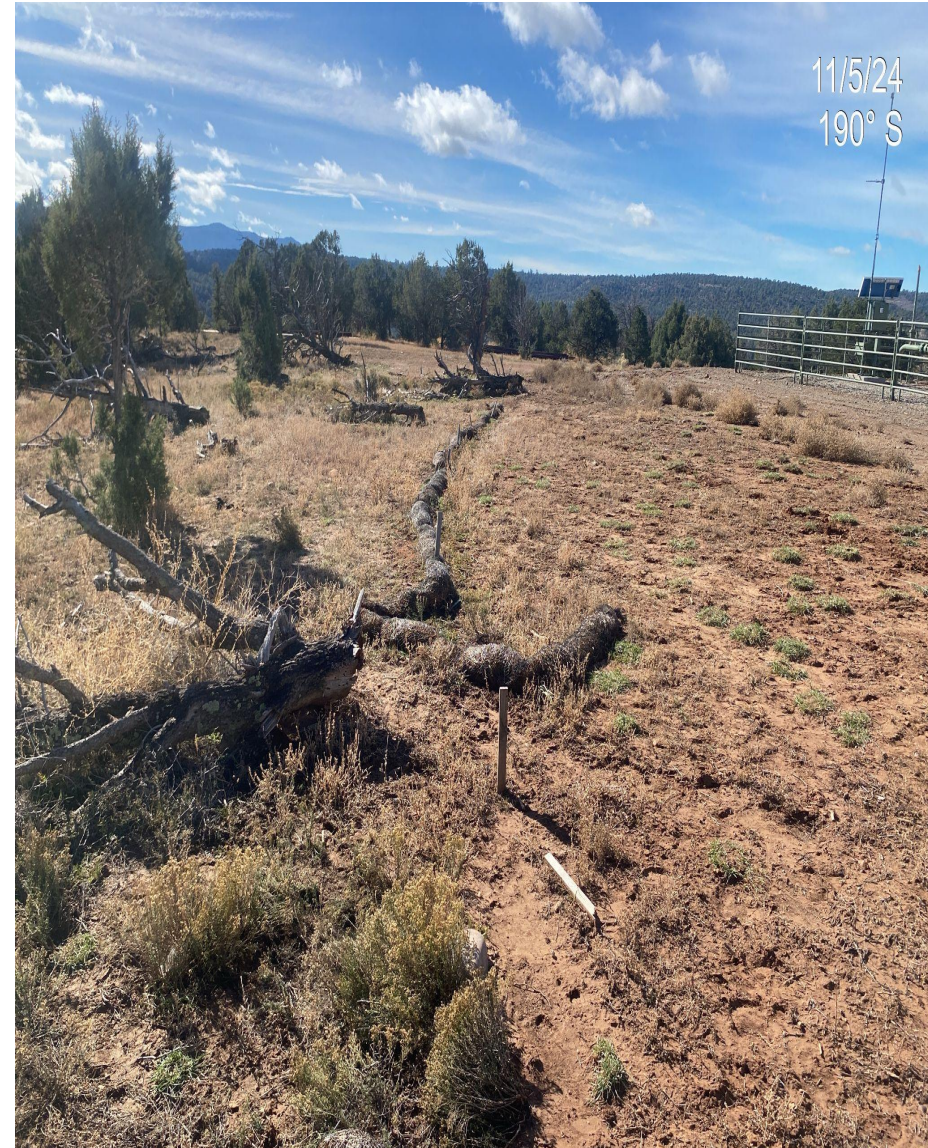
Photo 4. View of perimeter stormwater BMPs/wattles that are not installed correctly and no longer functioning. Determine if stormwater BMPs are needed if not wattles are considered debris and need to be removed.
