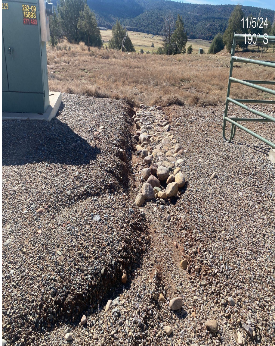
Photo 2. View of erosion forming along existing stormwater BMPs in the southern portion of the pad. Round river rock is likely contributing to formation of erosion.
