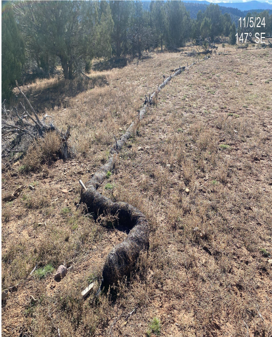
Photo 4. View of perimeter stormwater BMPs/wattles that are not installed correctly and no longer functioning. Determine if stormwater BMPs are needed if not wattles are considered debris and need to be removed.
