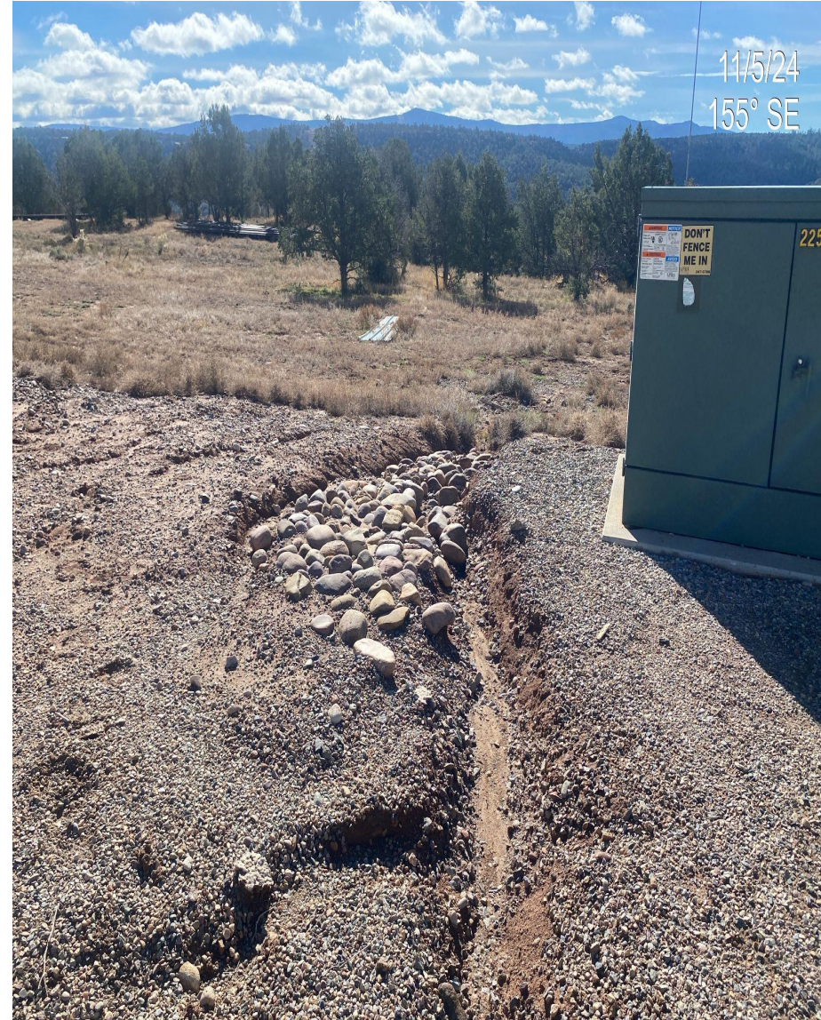
Photo 2. View of erosion forming along existing stormwater BMPs in the southern portion of the pad. Round river rock is likely contributing to formation of erosion.
