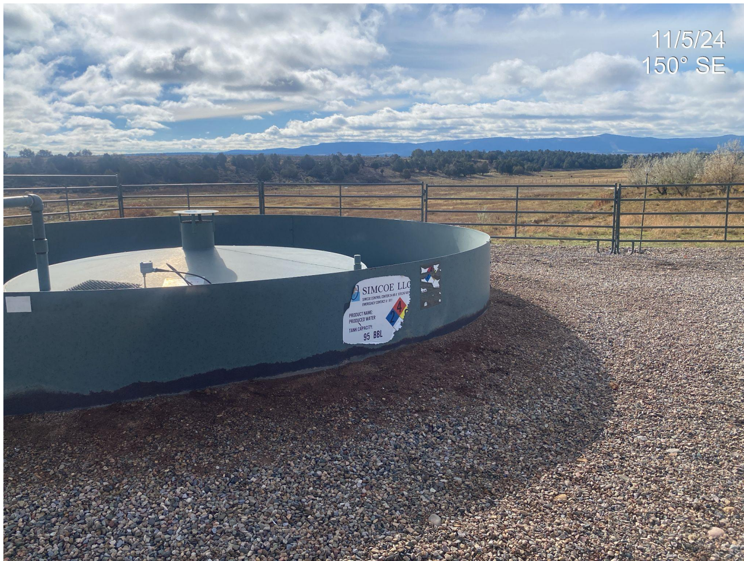
Photo 6. Produced water tank signs is starting to deteriorate.
