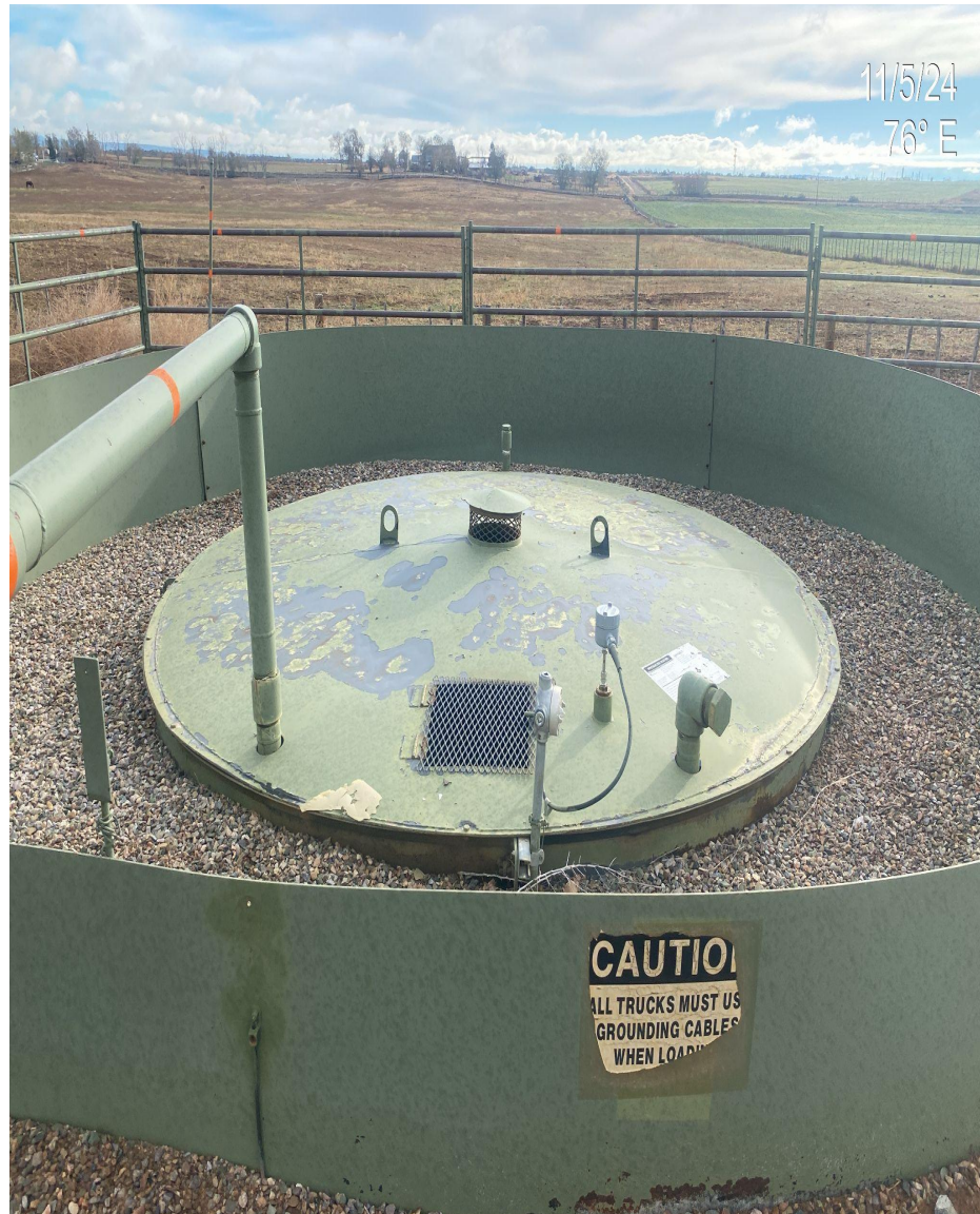
Photo 3. Produced water tank signs are deteriorating and no longer legible.
