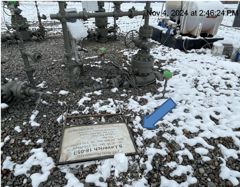
Photo # 8995 Wellhead sign laying on ground/not properly posted
