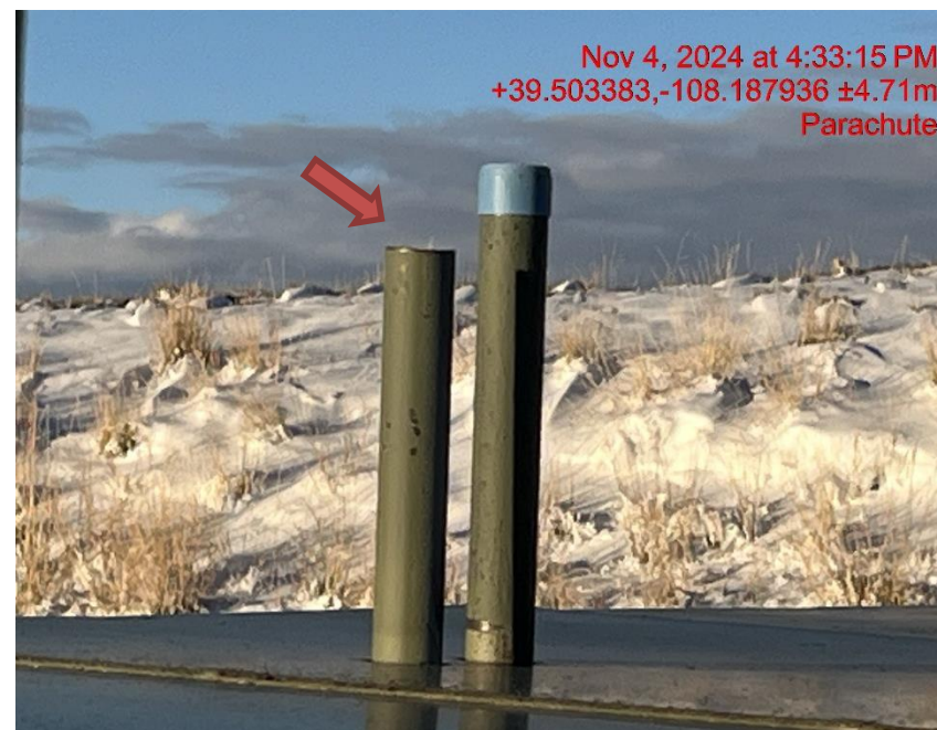
Photo # 8701 PRV vent line does not comply with CECMC pressure safety device rules
