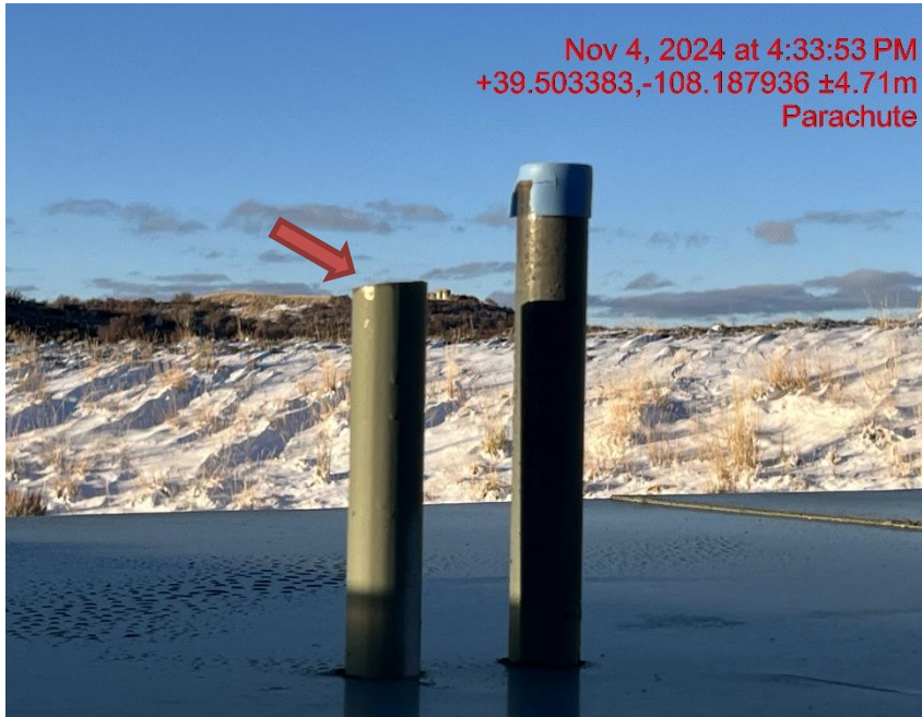
Photo # 8703 PRV vent line does not comply with CECMC pressure safety device rules
