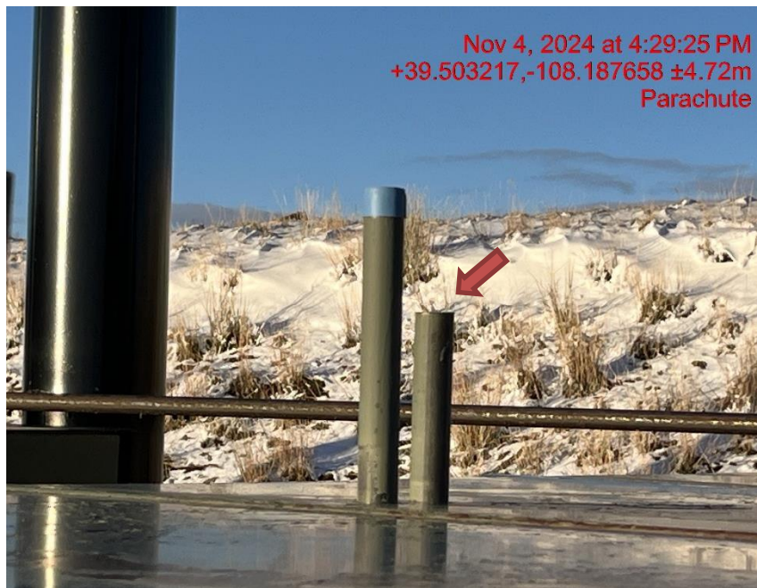
Photo # 8695 PRV vent line does not comply with CECMC pressure safety device rules
