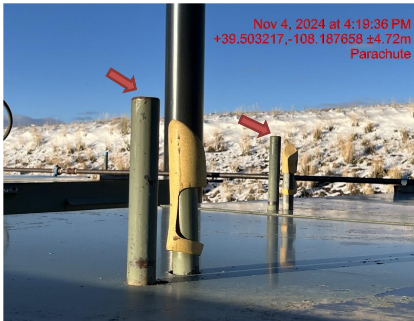
Photo # 8680 Rupture disc vent lines do not comply with CECMC pressure safety
