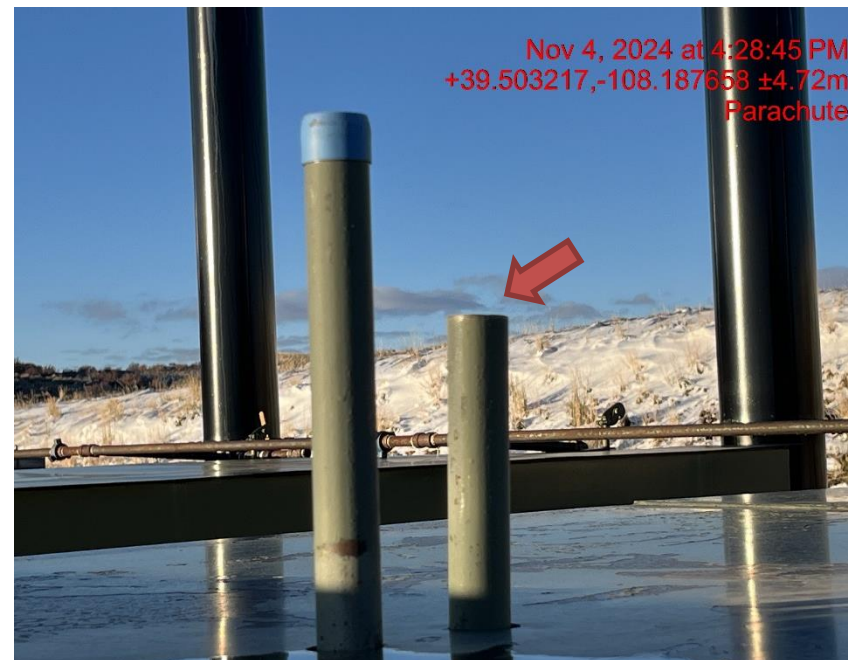
Photo # 8693 PRV vent line does not comply with CECMC pressure safety device rules
