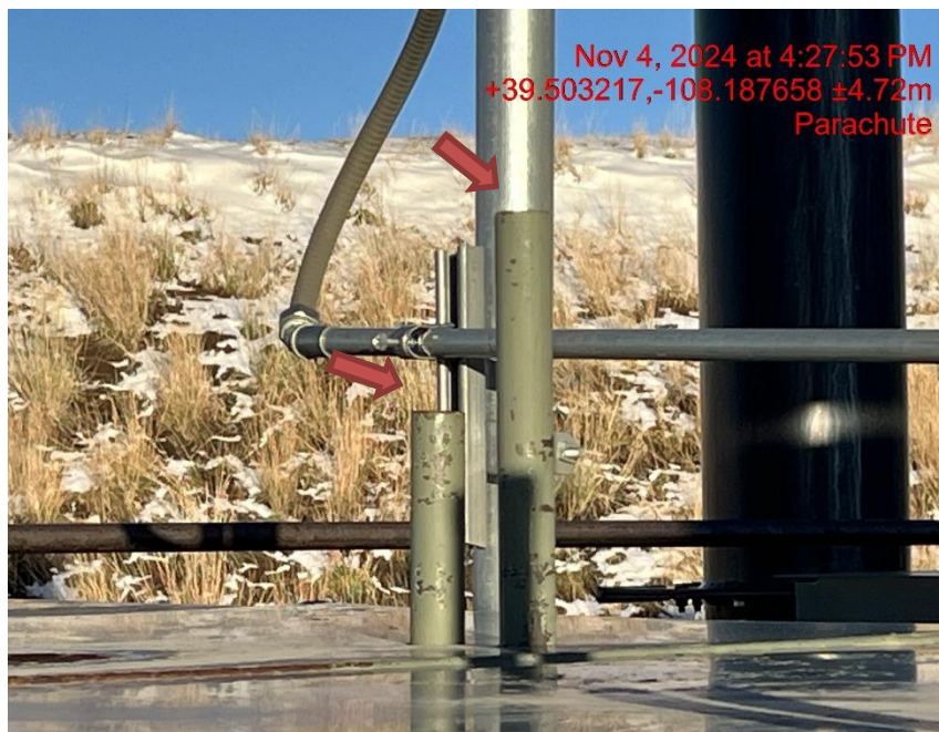
Photo # 8691 PRV & Rupture disc vent line do not comply with CECMC pressure safety device rules
