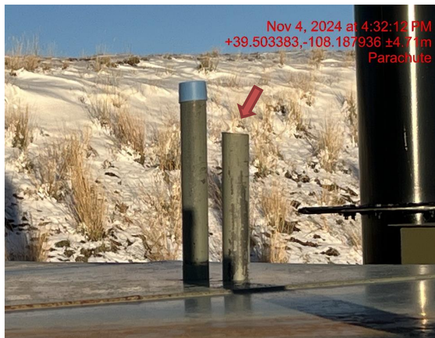
Photo # 8699 PRV vent line does not comply with CECMC pressure safety device rules
