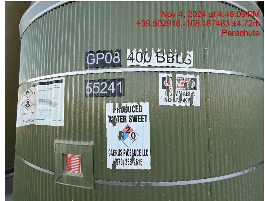
Photo # 8723 Tank labels damaged and illegible
