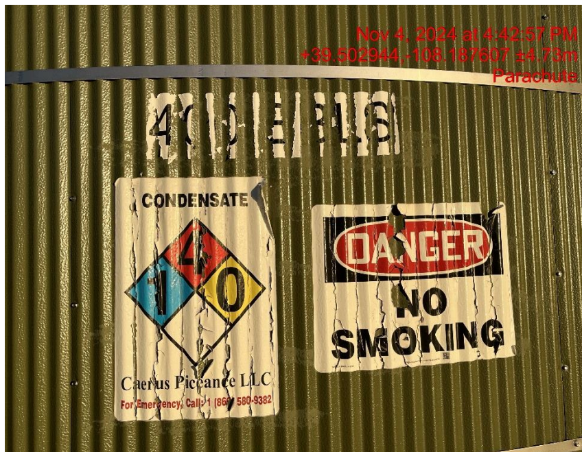
Photo # 8715 Tank labels damaged and illegible
