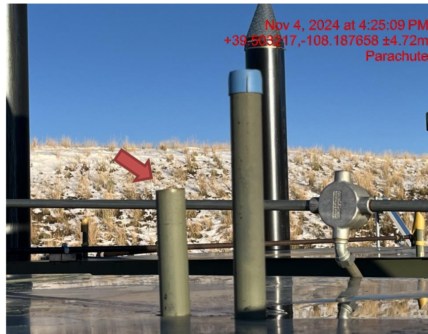
Photo # 8688 PRV vent line does not comply with CECMC pressure safety device rules
