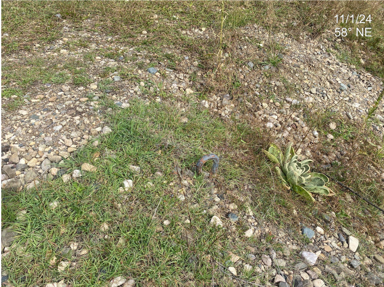
Photo 3. Unmarked guy line anchor in southern portion of the disturbance.
