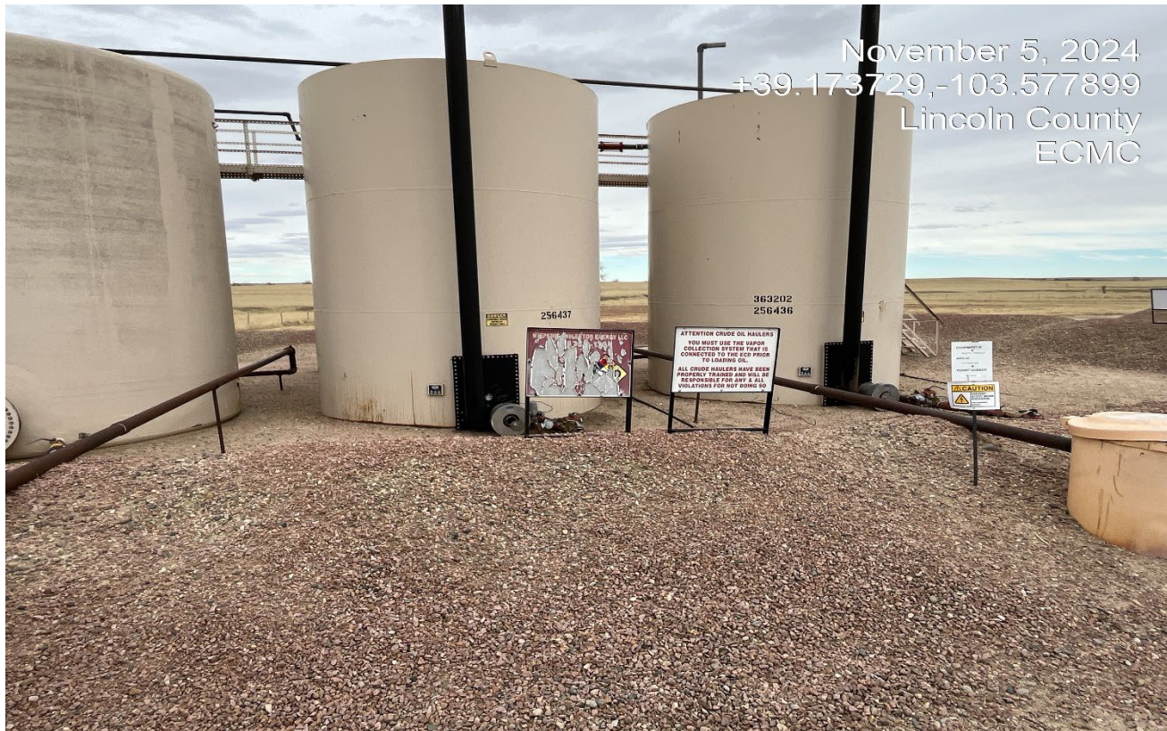
Photo 2. The sign at the tank battery is faded and needs to be replaced.
