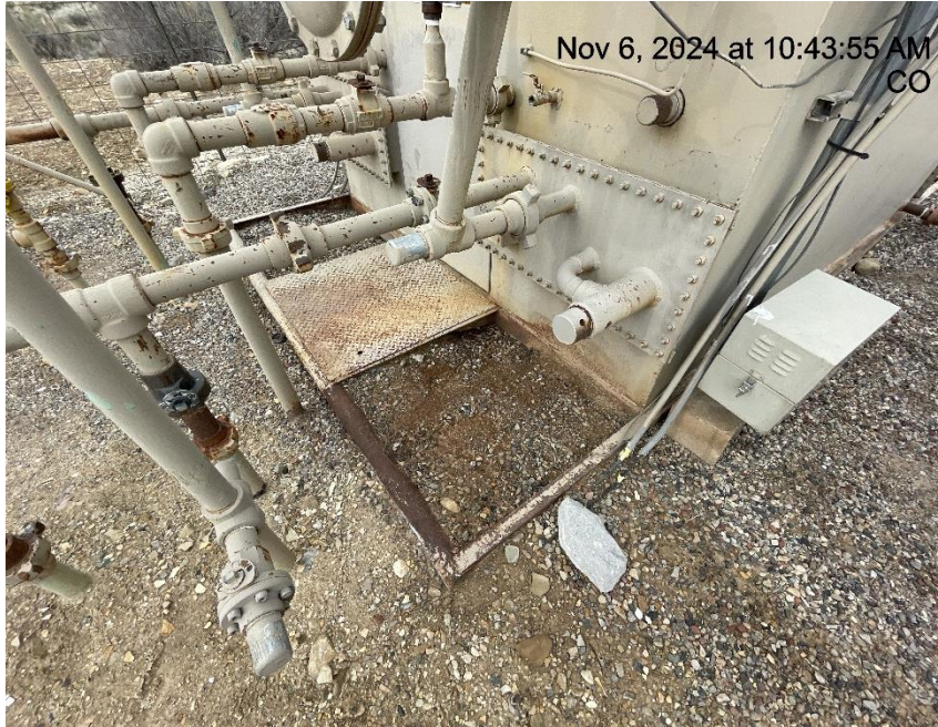
Photo # 9250 Staining near separator unit
