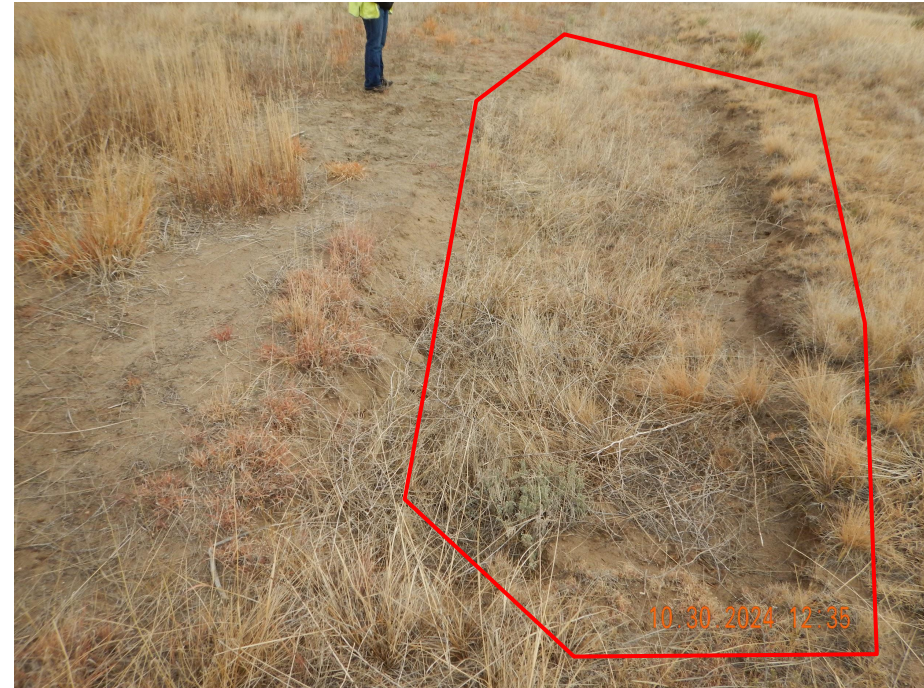
Photo 6. Photo taken from a portion of eastern access road just west of the location, facing East. Photo illustrates a portion of the access road that was not properly recontoured with evidence of historic erosion. Given the proximity to surface water (creek drainage), this shall be recontoured and long-term stabilization through revegetation.
